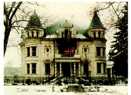
The Kearns Mansion, during and after the fire. The Christmas tree stood in the Grand Hall; the ceiling well, which had acted as a chimney, was closed in the restoration.
