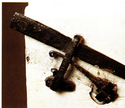
The rattle latch on the back door is original to the house's 1723 construction, most likely made by the house's namesake blacksmith. ABOVE: Front door and exterior shutters are painted sky blue.
