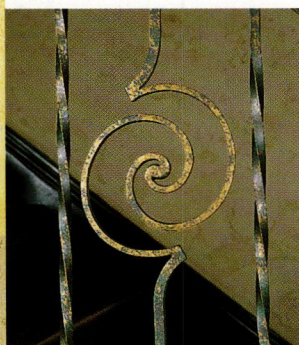
TOP: An original niche in the dining room holds a bronze coffee urn. LEFT: The wrought-iron stair railings were laboriously hand-stripped, uncovering their original patina. BOTTOM LEFT: A heavily carved Spanish Revival cabinet enhances the living room. Period wall sconces replaced missing fixtures. BELOW: The beamed dining-room ceiling is accented by original plaster masks; stenciling was added by the current owner.
