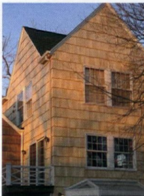
Eastern white cedar shingles, like these from Dow's Eastern White Shingles, look better on a "New Englander" than aluminum siding.
