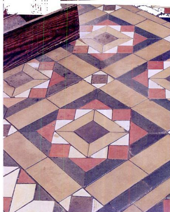
LEFT: Irresistible tiles in the style of Ernest Batchelder, by Tile Restoration Center. ABOVE: Salvaged tile? These encaustic floor tiles were painstakingly carried, cleaned, and relaid by a New York City homeowner, who got them from a local church demolition.
