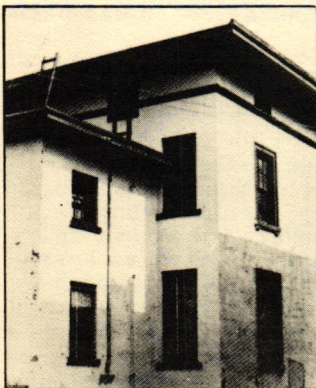
BEFORE renovation the Villa was a boarded-up derelict.
