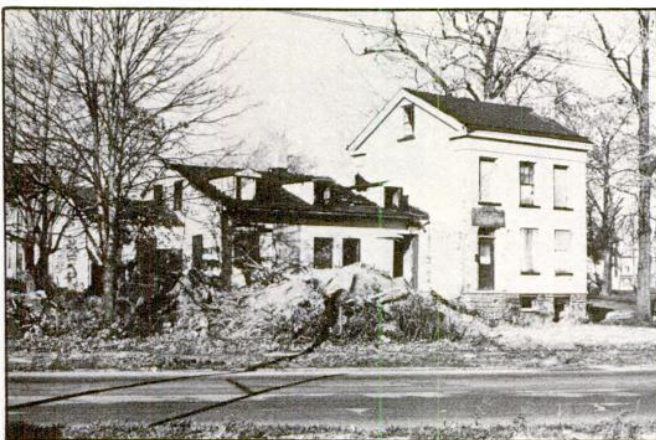
The house as it was on its original site. There had been no indication that the back wing was an addition until it began to move away from the house when it was lifted onto the wheels.
