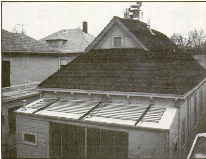
Heat collection coil is tucked on a back porch roof where it doesn't affect the appearance of the house. Aluminum paint on roof reflects heat back up to the black painted pipes.
