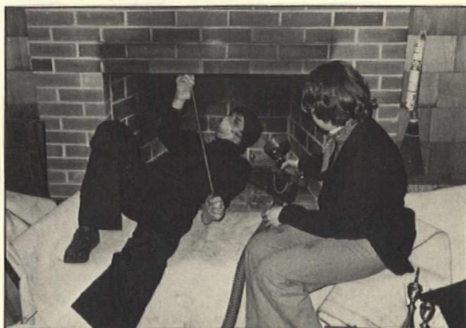
Eva Horton is cleaning the smoke shelf with a special brush. You can use an ordinary broom, but don't forget the face mask. Her assistant holds the flashlight.
