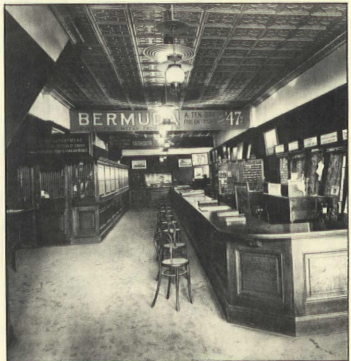
A typical commercial installation of tin ceiling in the New York office of Thomas Cook and Son travel agency, c. 1906.
