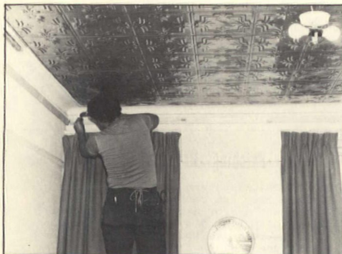
7. Next, furring strips are nailed to wall for the cornice. When smaller metal cornices are used, it usually is nailed directly to the wall.
