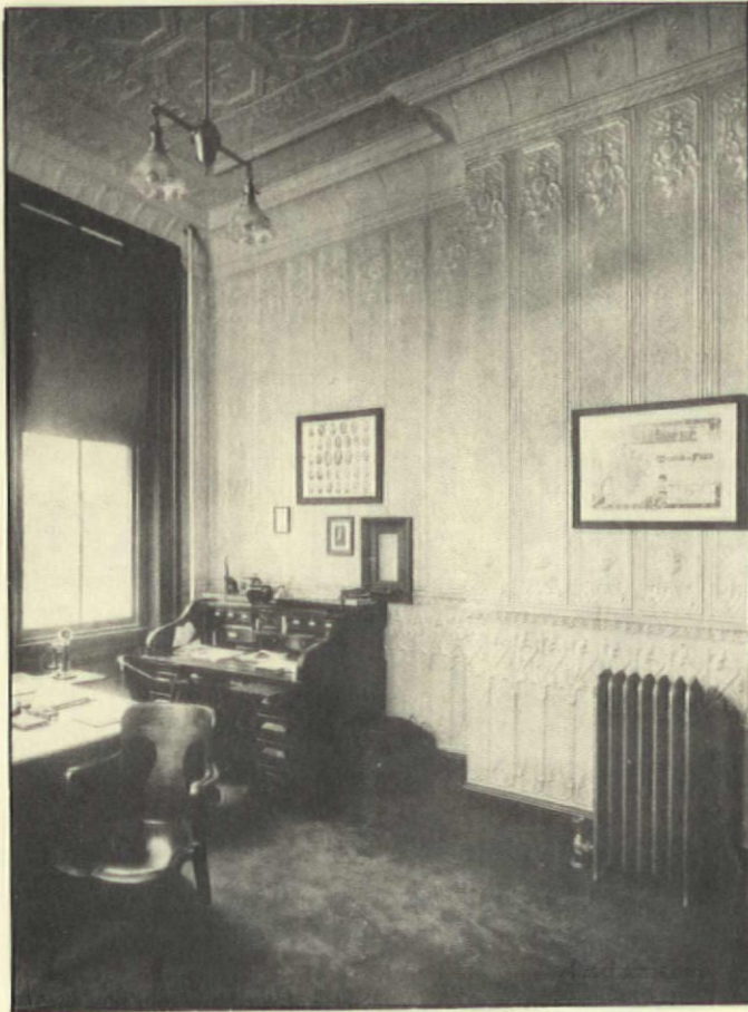
This photo of an office was featured in a turn-of-the-century steel ceiling catalog. Ceiling, cornice, walls, and dado are all covered with various forms of metal sheets.
