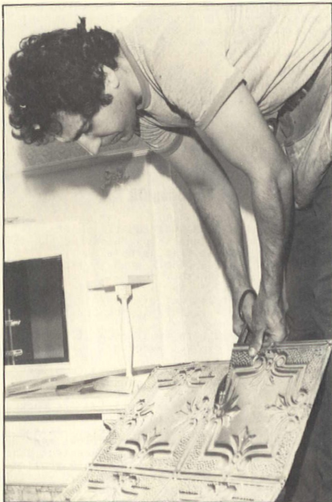
6. When metal panels need to be cut, such as at the edges and corners, job can be done with tinsnips. Beware of edges: They can be razor sharp!
