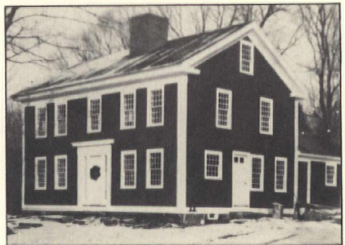
After restoration--the clapboards are now painted brick red as they were originally.
