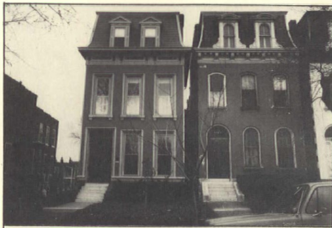
This photo shows the Keay home after completion of the third storey addition.
