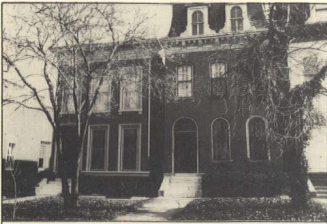
The Keay home is on the left, shown prior to reconstruction of the third floor.
