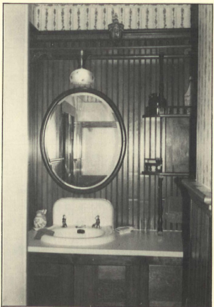
In this view, the wainscoting and two-part cap moulding can be seen at right.
