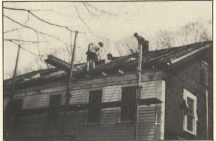
During the roof restoration the original hand-hewn rafters were reinforced.
