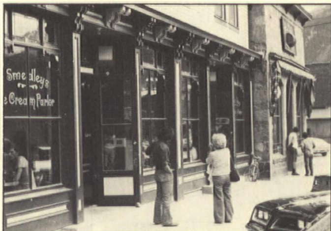
The Victorian effect of this store is achieved by attention to every detail including: Art glass in transom windows, two kinds of brackets and multi-color paint job.
