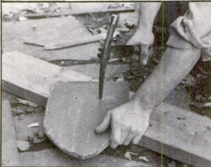
RIPPER: Cast-steel tool 24 in. long used for removing damaged slate. Thin blade is slipped under broken slate and hooked around nail shaft. The other end of tool is struck sharply with a hammer; end hook cuts and withdraws the nail. (left)
