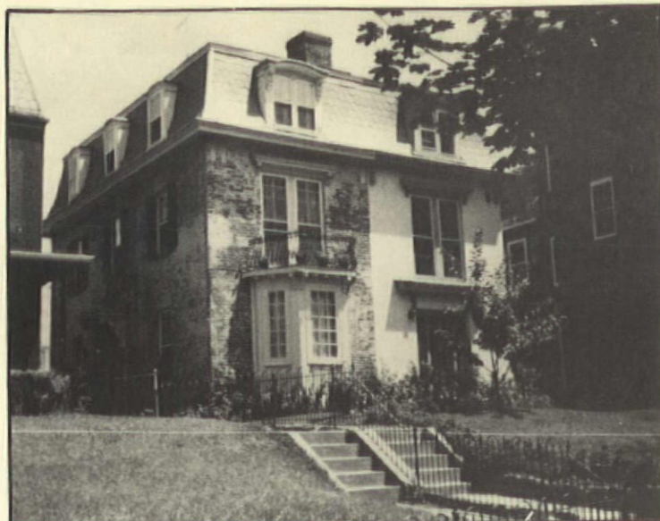
THE HOUSE RESTORED, 1979. Mr. Giordano is hand-scraping the brick to gradually remove paint.
