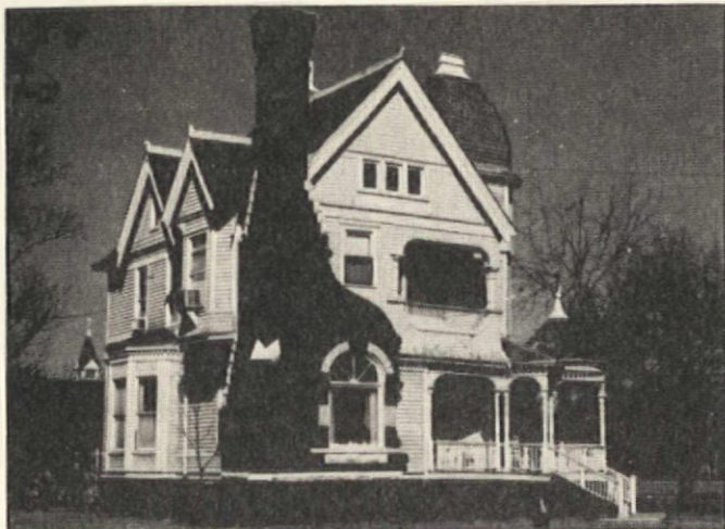
The Parrish House in Calvert, Texas was used as an example of Queen Anne style in Marcus Whiffen's well-known architectural style-book. It is being restored to c. 1890 by its present owner.
