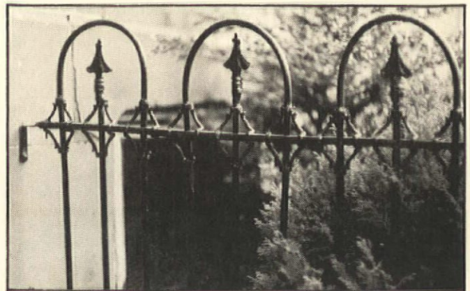
A typical hairpin style fence, welded up by the author from new steel and old cast-iron fence parts.
