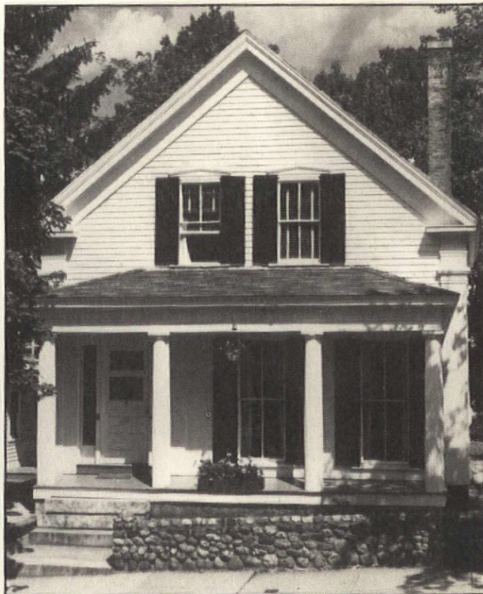
This is the house after exterior restoration. Note the removal of the second-floor bathroom window. (Photograph by Tony Schneider.)
