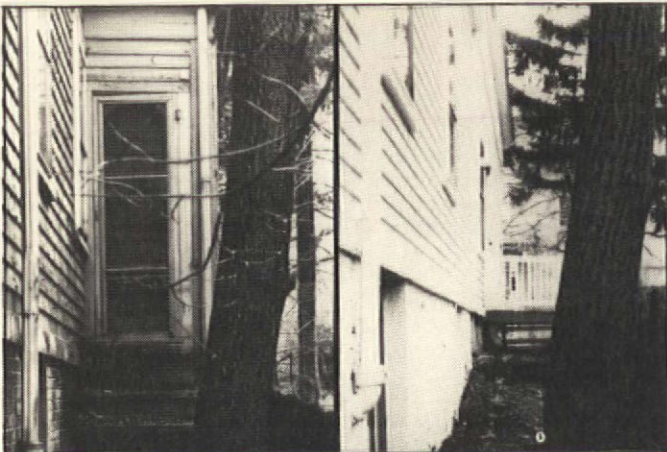
The kitchen addition, pictured left, was not part of the original house. It would have been kept, but its poor construction and maintenance rendered it unsalvageable.
