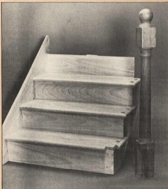
This shows a connection detail for the main (bottom) newel. The base of the solid newel has been housed to receive the tread, riser, and string.
