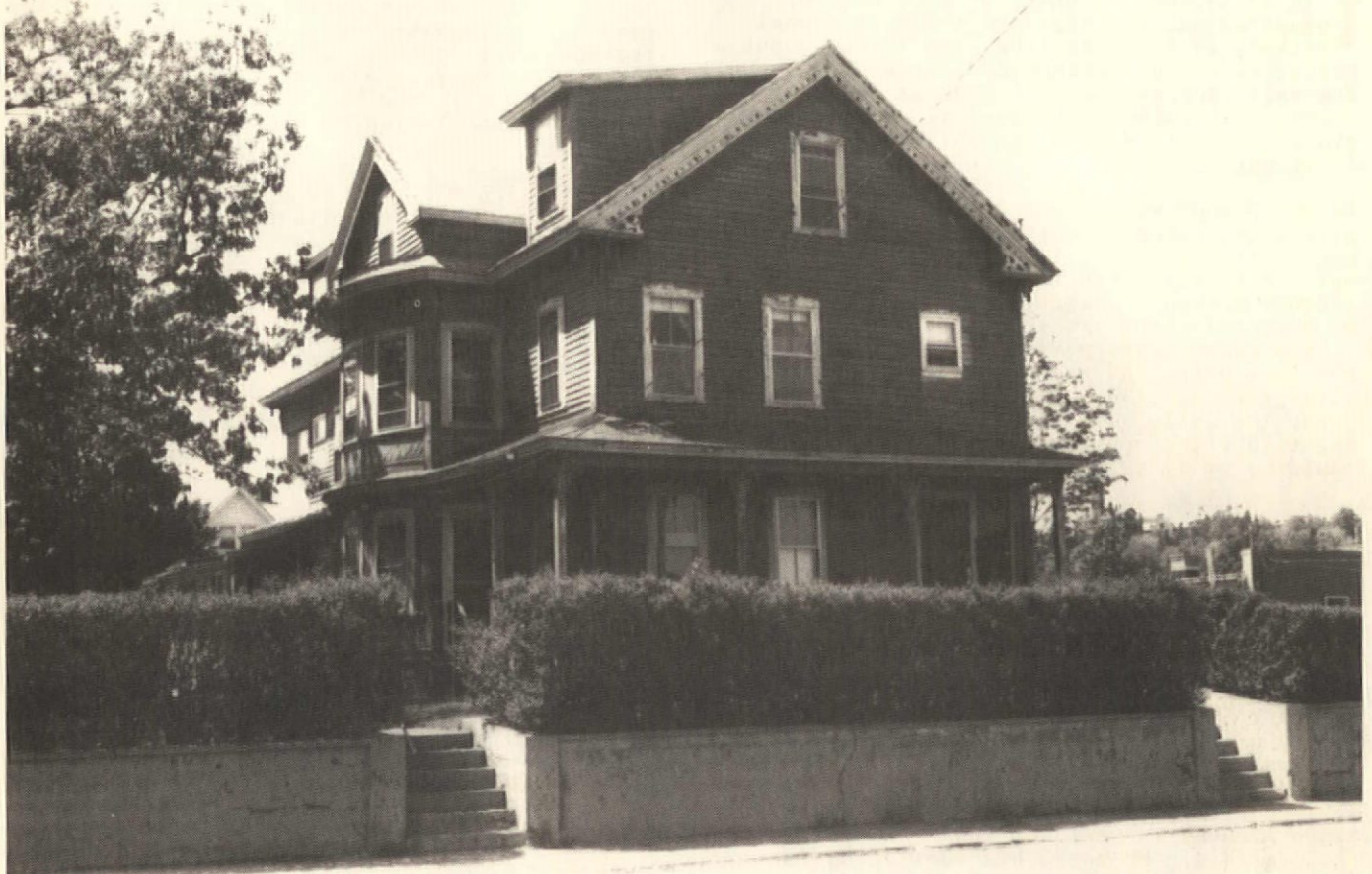
This post-Victorian house, if not regarded with the necessary sensitivity, could eventually suffer the harshest of renewals.
