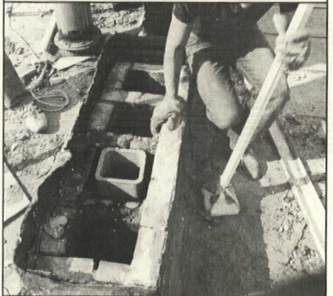
Above: This section of clay liner has been buttered with refractory mortar. It will be lowered onto another, similarly coated section, and will have another section lowered onto it. Below: In this photo, you can see that the chimney stack has four flues, only one of which is being lined.
