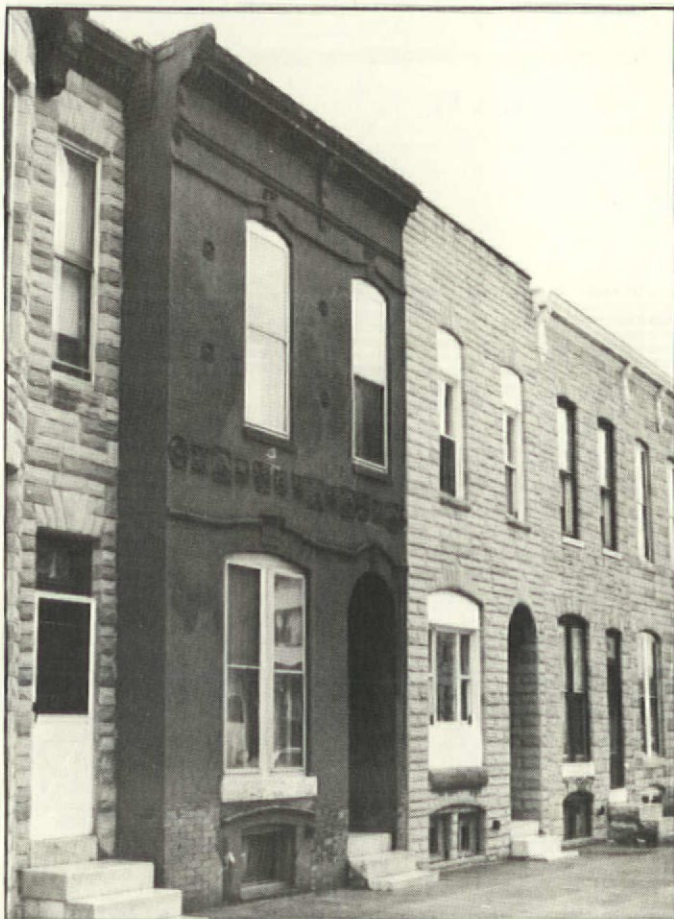
It's most likely that, before Formstone, the house on the right had a cornice, windows, and terra-cotta ornamentation just like the painted house on the left.
