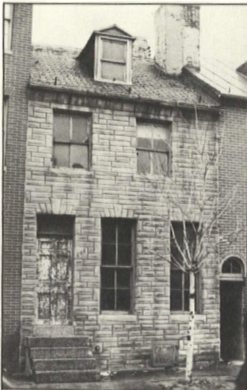
Close to half the Formstone facade was removed in only 4 hours.
