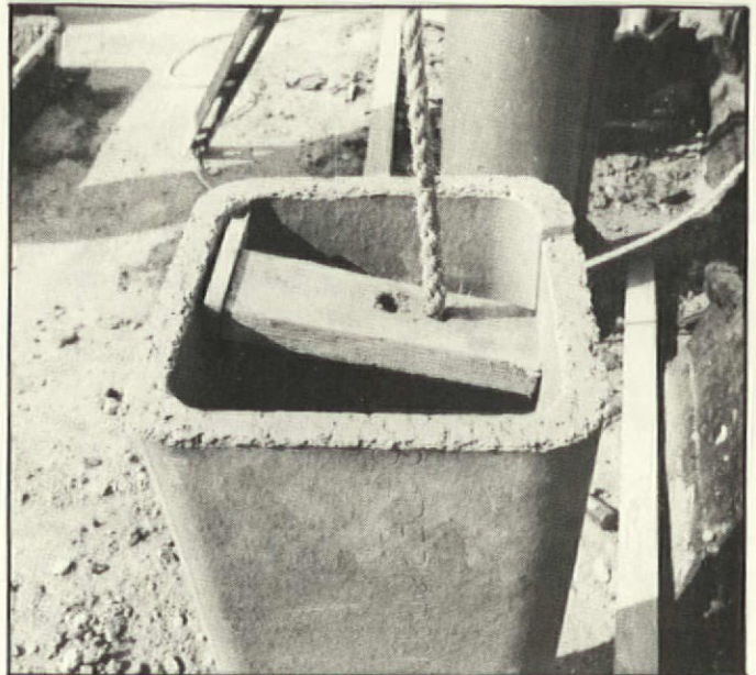
Above: This section of clay liner has been buttered with refractory mortar. It will be lowered onto another, similarly coated section, and will have another section lowered onto it. Below: In this photo, you can see that the chimney stack has four flues, only one of which is being lined.
