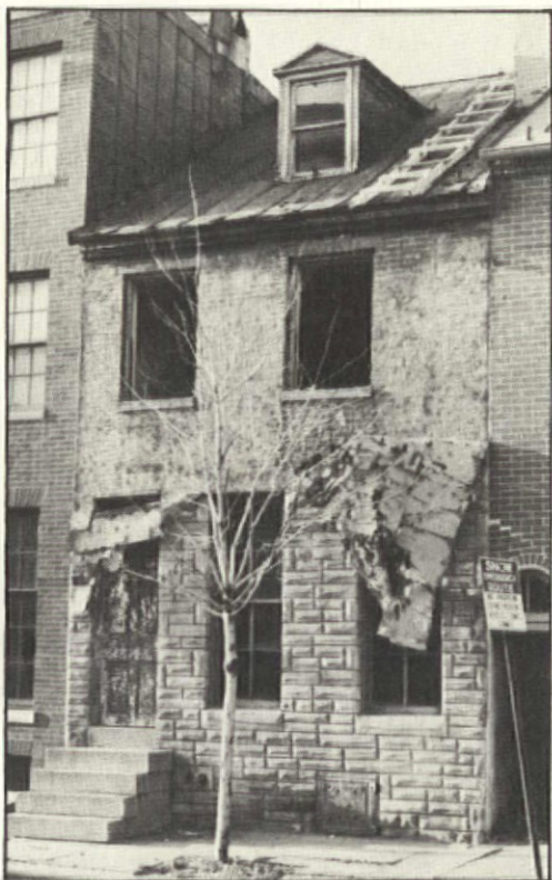
Close to half the Formstone facade was removed in only 4 hours.
