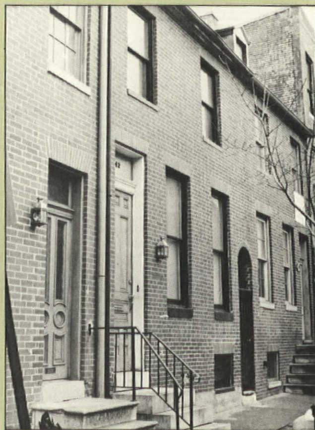
Above: The Formstone is off, the mortar joints have been cut back slightly, and the brick has been cleaned. If the job has been done properly, this is about as bad as the brick will look. Right: All three of these circa 1840 Federal rowhouses were once Formstoned. And unless you get really close, the bricks look fine, don't they?
