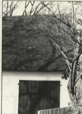
A butt-end view not usually apparent. Actually, color, size, ridges and eaves are all good wood simulations on these new concrete tiles.
