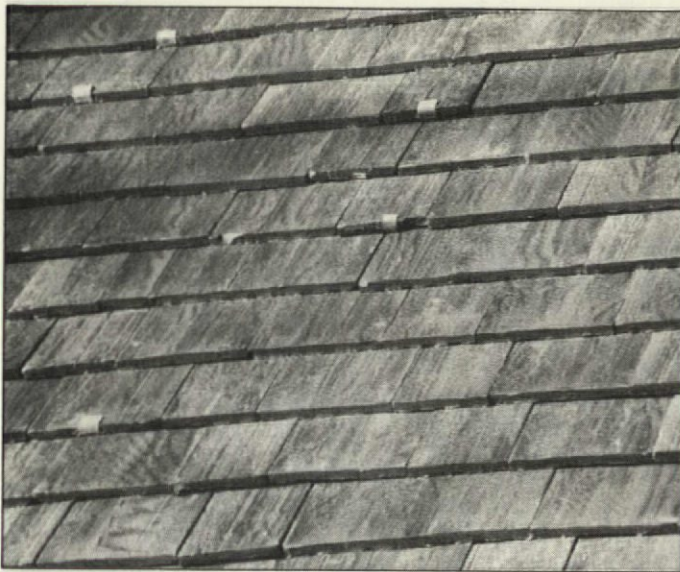
Even up close, square-butte clay tiles are admirable wood stand-ins. But all broken tiles show tell-tale red. Tabs hold replacements.
