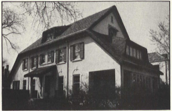
mers, and the varied bays and oriels. From the Jacobean era come the overall symmetrical organization of the house and its massive brick gable ends with decorative stone parapets and ball finials. The house at right is a Cotswold Cottage designed by Mayo in 1919. Its plain stucco walls, shed roofs, rounded eaves, and hooded dormer suggest that Maid Marion might beckon Robin Hood from the porch.
