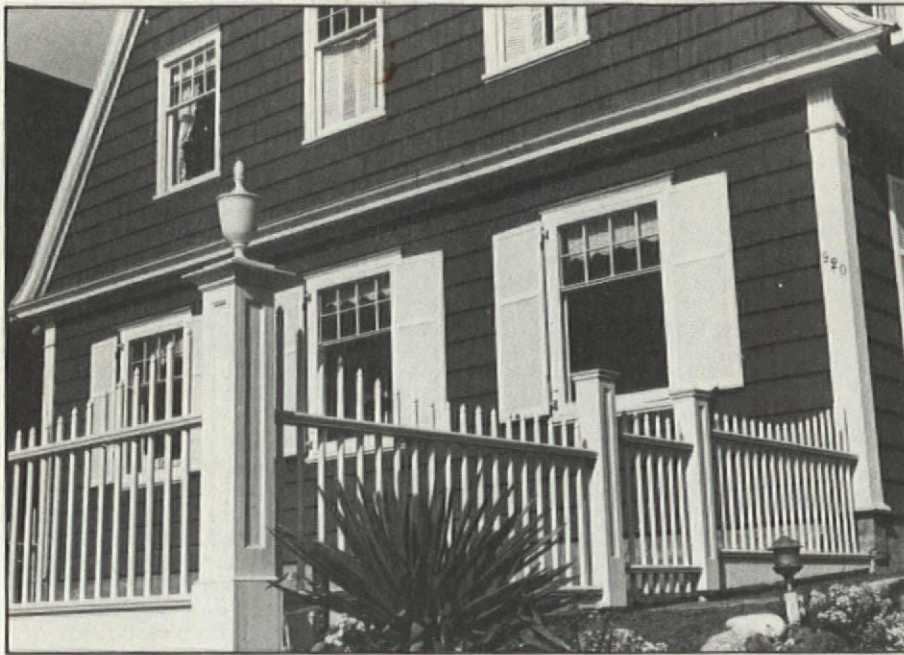
The new fence echoes the architectural detailing of the house. Notice the similarity of the pilasters and fence posts, the sweep of the pickets and curve of the roof. Stair stepping of the fence and good ground clearance are all construction details worth noting.
