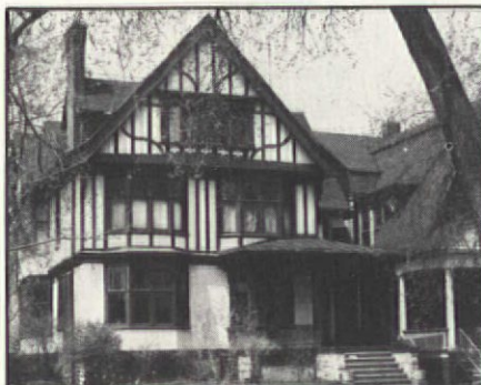
Ernest Mayo's design for this 1894 Evanston residence includes Arts and Crafts detail on an essentially vertical American Queen Anne. The half-timbering, two-storey window bays, and porch with Tudor archways are preludes to the full-blown English Revival. Note touches that suggest "craftsmanship": the curvilinear bracing in the gable and trefoil panels below in the attic windows.
