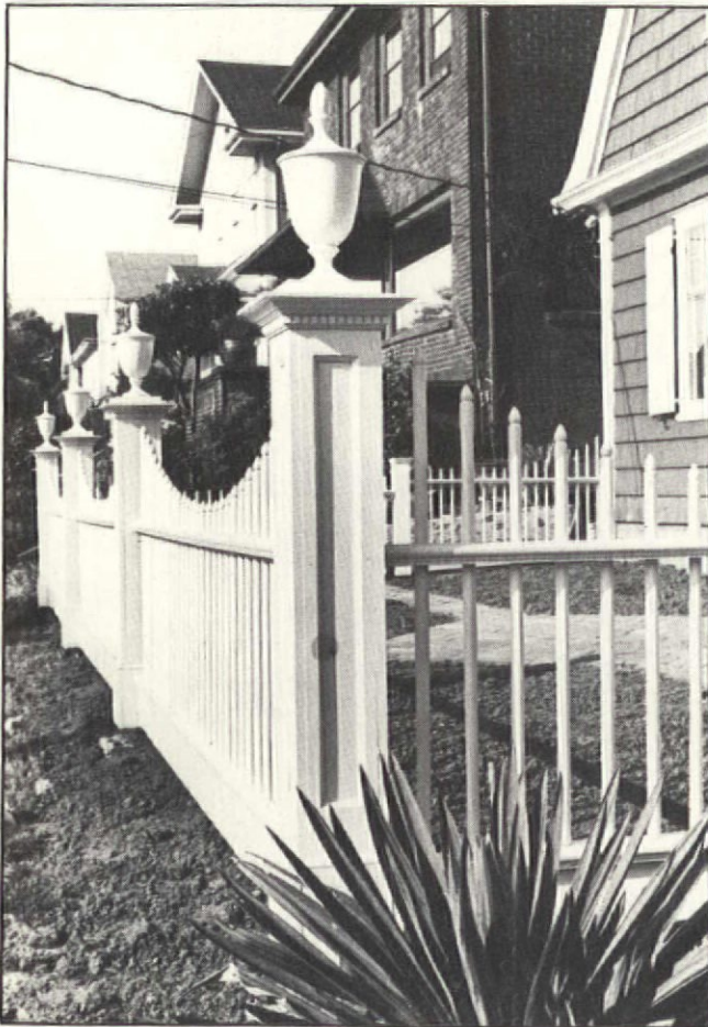
A gentle, dipping, curved effect is created by varying the picket lengths, similar to the more complicated ramped top rails seen on some early fences.
