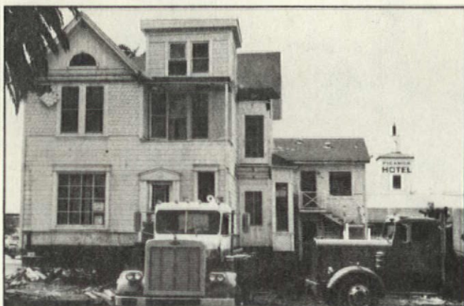
Above: The house has been raised and is ready to roll. Without the huge portico, it's now starting to look more attractive. Below: The house is at its new site, and the real work has begun. The scaffolding was needed for the stripping of the old paint, as well as for the imminent attachment of the tower roof. That's it sitting in the grass, like a little pyramid. Alan and LaDel built it themselves in just a few days, copying it from old photos of the house. A shingler finished it up, the crane arrived, and 30 minutes later the tower had a roof once again.
