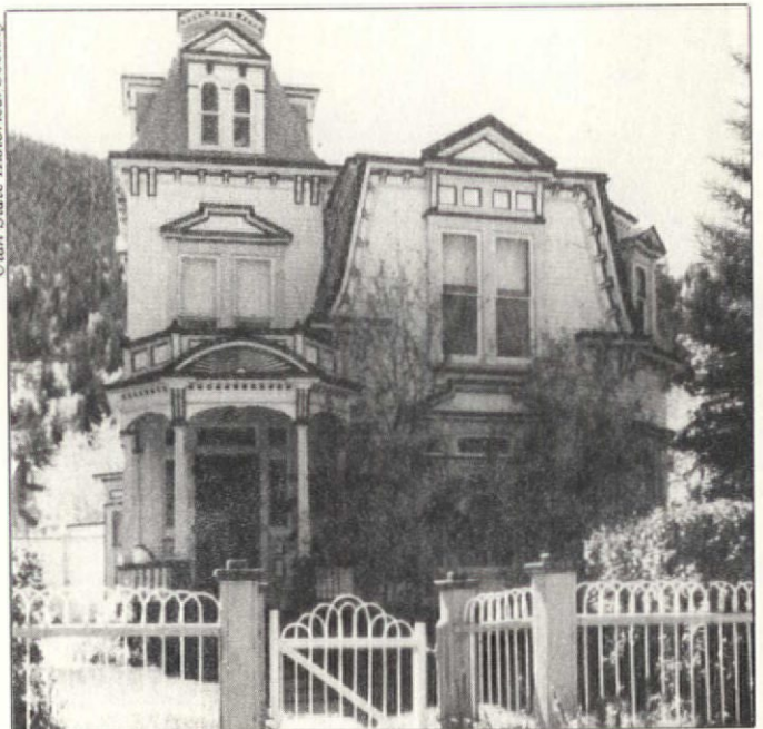
A grand, polychromed mansardic house in Georgetown, Colorado.
