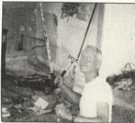
Bob Kay (a.k.a. "Pa") repairing a crawlspace.
