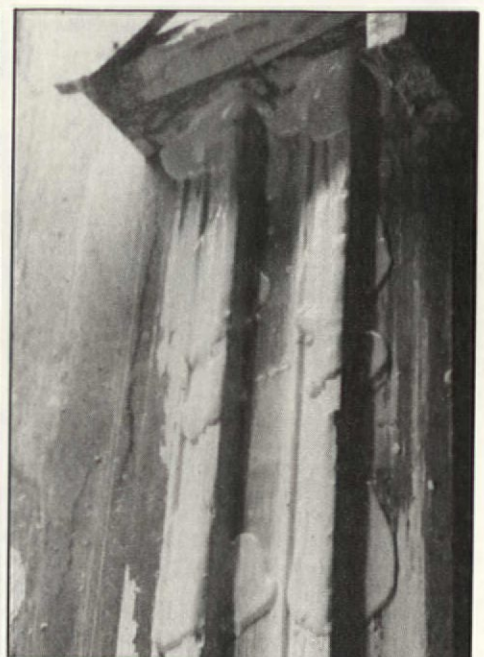
Step 7: Dab plaster on gaps in the moulding and run the mould over them.
