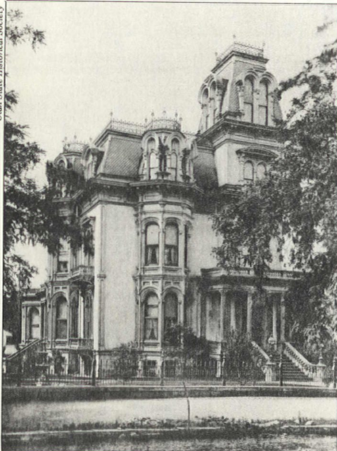
A perfect example of the American Second Empire, the Gardo House in Salt Lake City was razed to make room for a bank.
