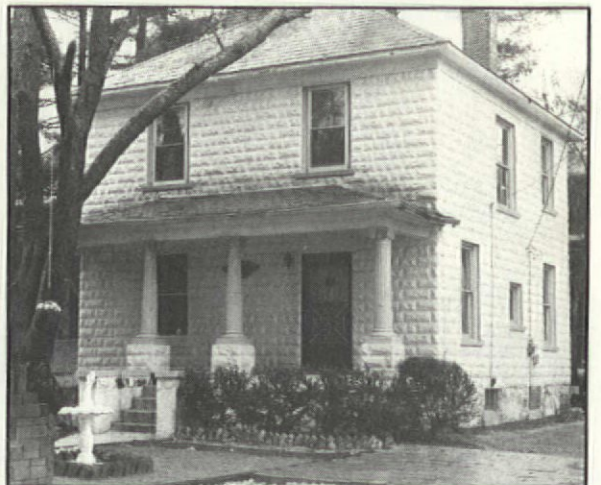
The American Foursquare came dressed in shingles, clapboards, stucco — and cast concrete block.
