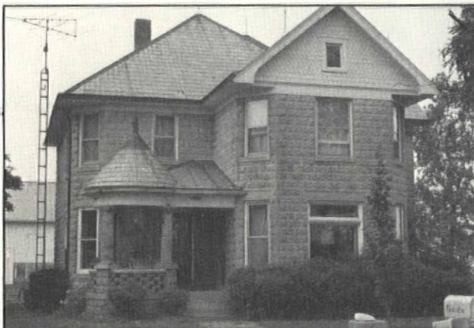
This concrete block house was built in 1912, but it has many elements of the Victorian Queen Anne style. There are some examples of cast block used in late Victorian-era buildings — but not many.
