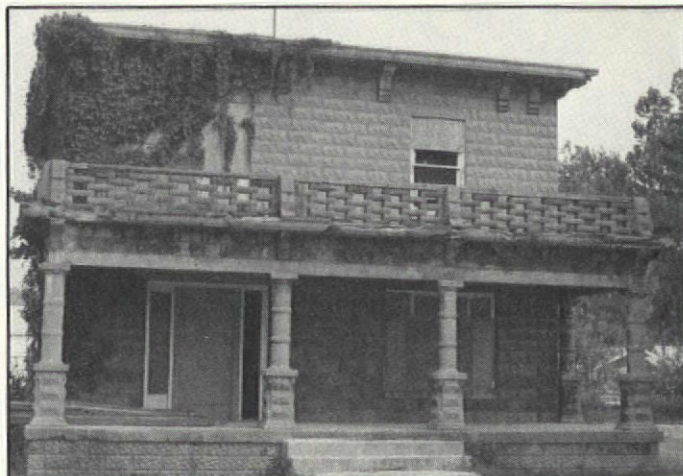
Columbus, Indiana, circa 1915: A handsome concrete house built on the common foursquare plan. Note cobblestone-face blocks in the foundation; brackets and columns are cast, too.
