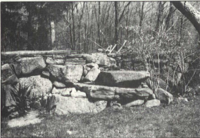
Above: This isn't just some pile of rocks; it's an 'upping stone,' and is most likely original to the house. The rocks are arranged in a stepwise fashion so ladies could climb onto horses or into carriages without abandoning any of the demeanor that made them ladies in the first place.
