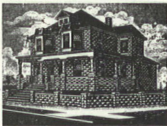
House, porch columns, balustrade and retaining wall all built of Hollow Concrete Building Blocks.
