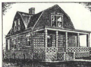
A Cottage built of Hollow Concrete Building Blocks.
