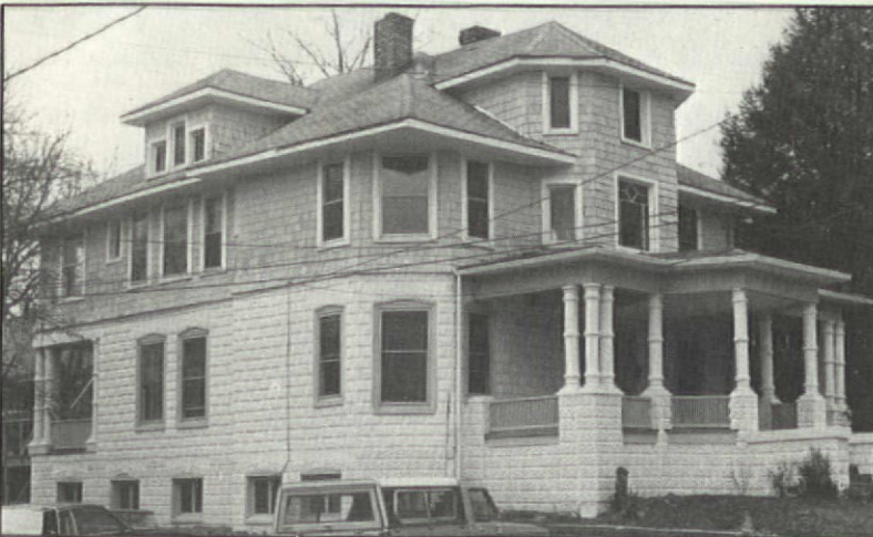
It was quite popular for houses to be built with a concrete-block foundation and porch, but a wood-frame upper storey finished with clapboards or shingles. The wood balustrade between piers is a variation on the all-concrete porch.
