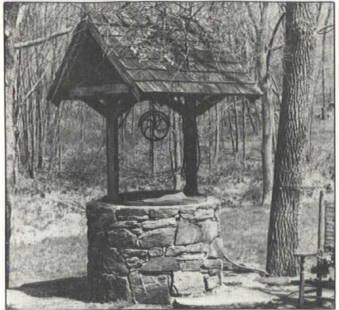
In the 1908 photograph on the opposite page, you can see the original Sterling Heights well: The diagonal pole at the center of the picture is part of a mechanism that two people had to operate. The well was also level with the ground, which is not the safest arrangement if you're raising children on the farm. Thus, when the Bakkes took over the property, they built the curbing seen here, added the little roof, and simplified the mechanism for drawing water.
