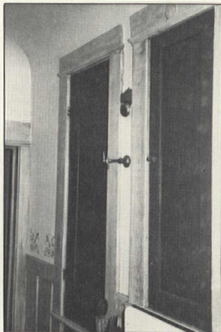
Coved ceilings are typical of early-20th-century homes. Note the gas jet and doorbell on the wall.
