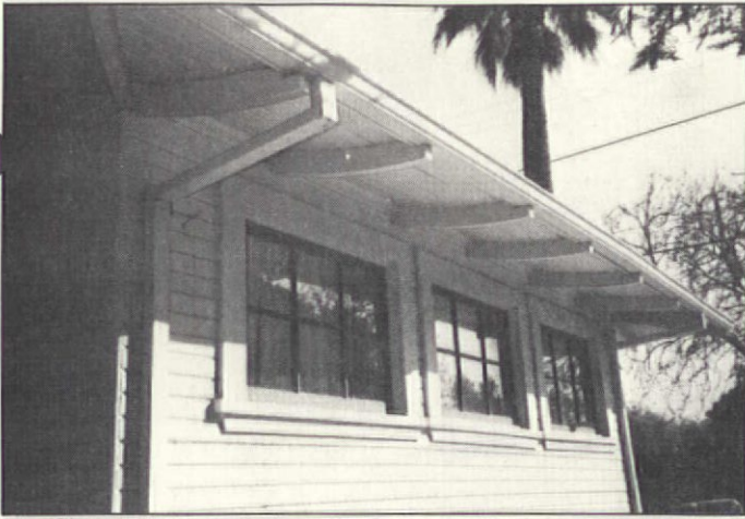
The sleeping porch, like the entire house, has Japanese-style rafter ends.
