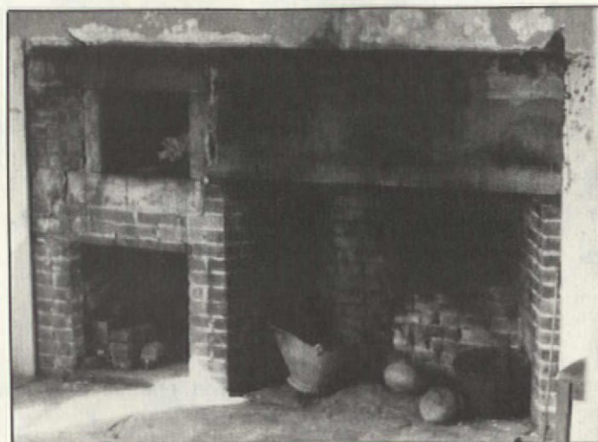
The bake oven in the ell as it appeared before the Conlons restored it.
