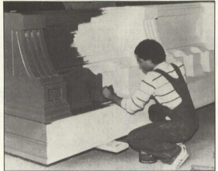
A proper paint job is essential for cornice longevity. If it's well designed and maintained, a shop-built cornice should outlast the building to which it's attached.
