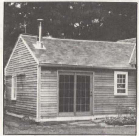
The carriage house was turned into a spacious kitchen. The Conlons made kitchen cabinets from the original oak-plank flooring.
