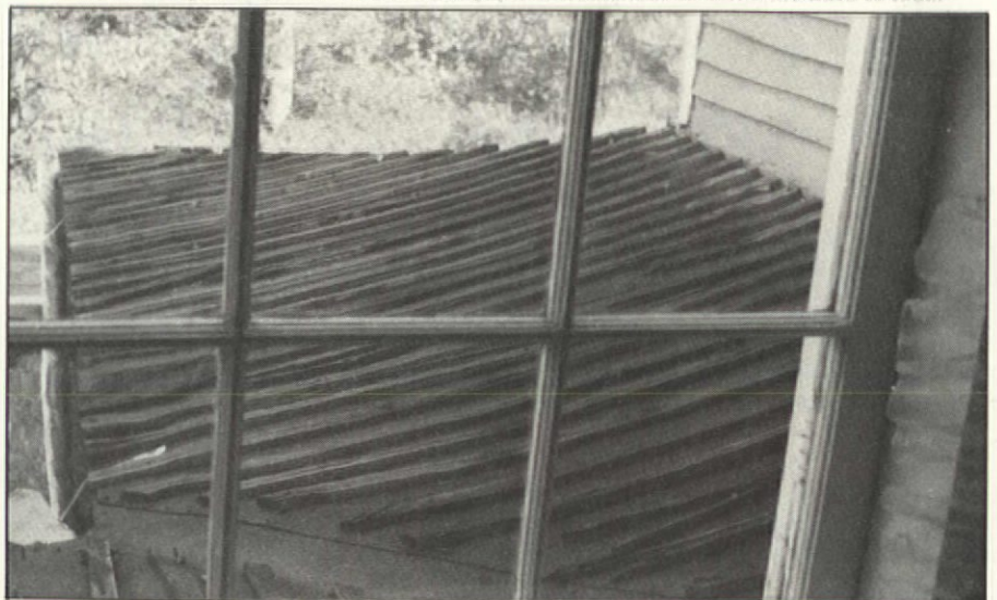
Left: The restful porch of Yesteryear House. Below: Originally, the porch had a board-and-batten roof. "The entire front porch was rebuilt in 1947, but it leaked badly. Dad covered it with roll roofing and replaced the batten strips, so it would look as it was intended to look."
