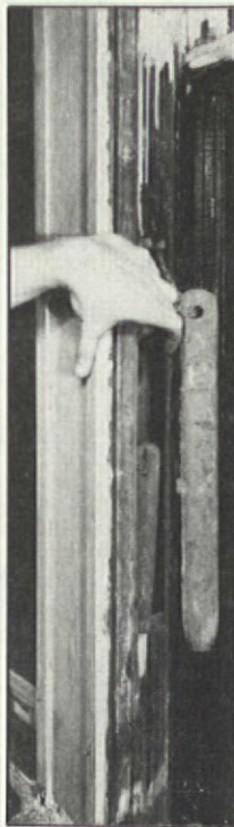
Counterweights are easily accessed through a panel in the jamb.
