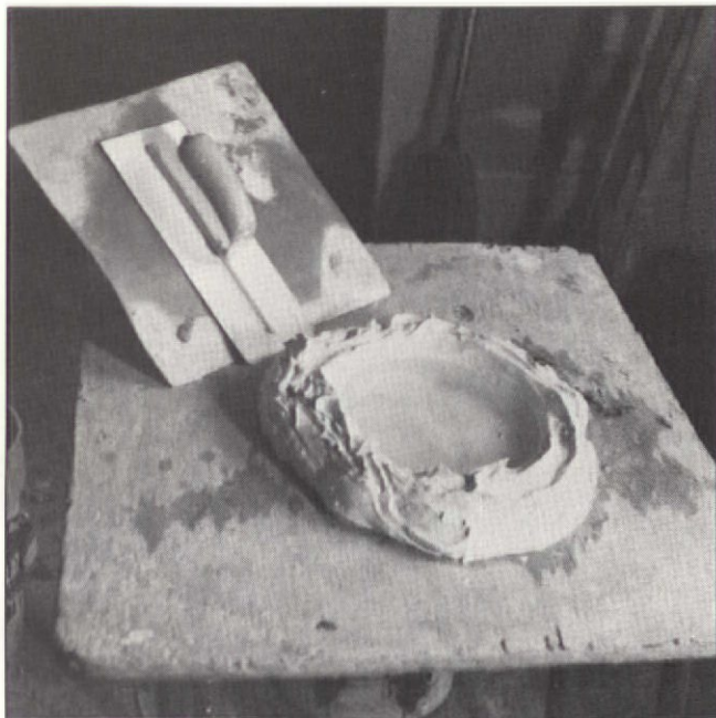
The lime putty ring on a mortarboard.
