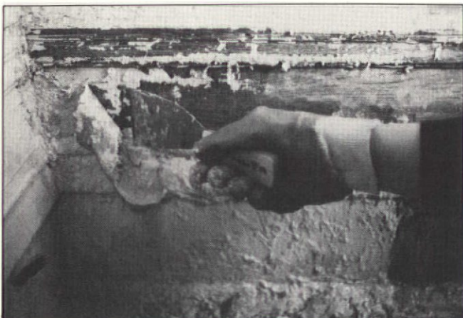
Hand-stripping assures excellent results. This photo demonstrates one of its drawbacks — the mess.
