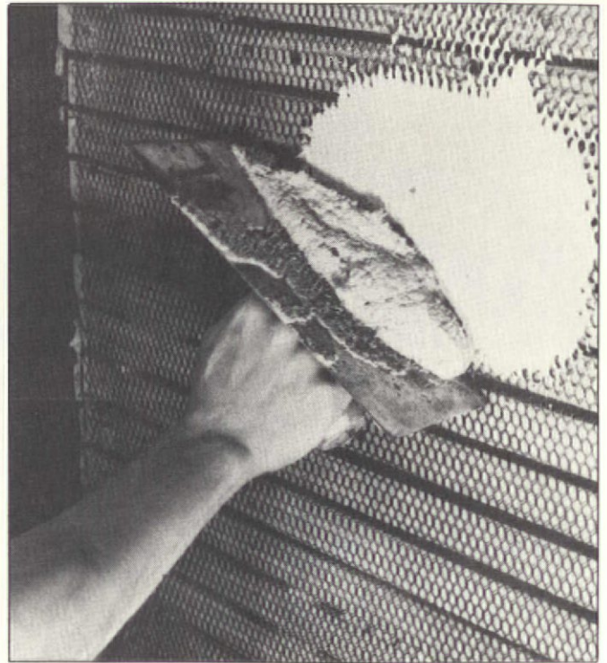
and applying it to the lath.
