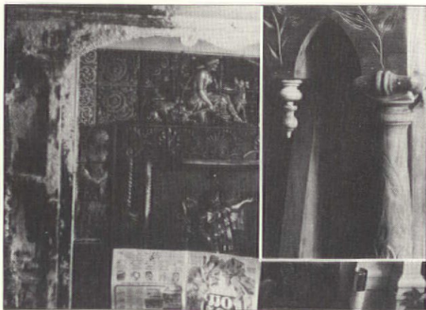
The library's spectacular fireplace, complete with embossed tiles, was carefully stripped of a coat of white paint.
