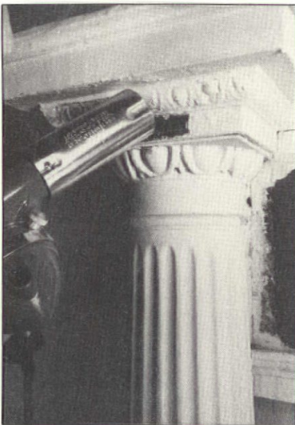
The HG-501 blows hot air into carvings — causing paint to melt. The tool is ideal for stripping ornamental woodwork, and will strip flat work as well.
