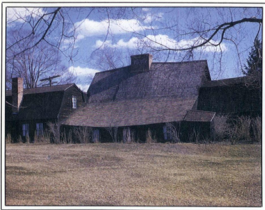
The Fairbanks House, Dedham, Massachusetts, was built in three sections, ca. 1637-ca. 1680. The steeply pitched roofline of the oldest, center portion extends across the lean-to at the rear of the house, reaching nearly to the ground.
