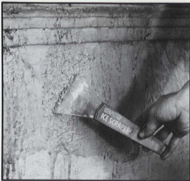
Marble again. This time, loosened paint layers are removed with a plastic ice scraper.
