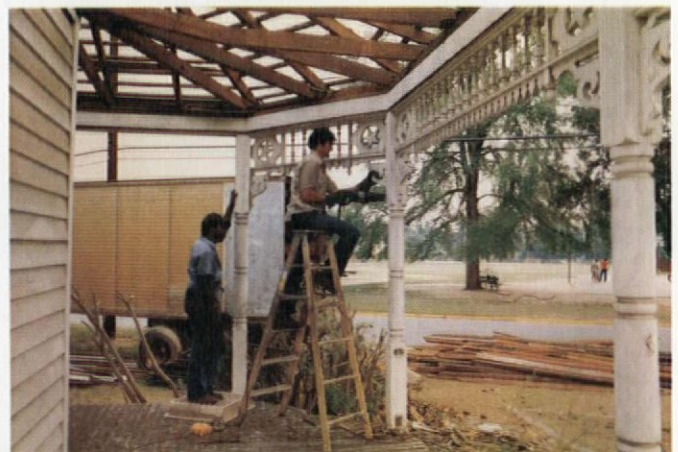
Bob removing fretwork from the front porch.
