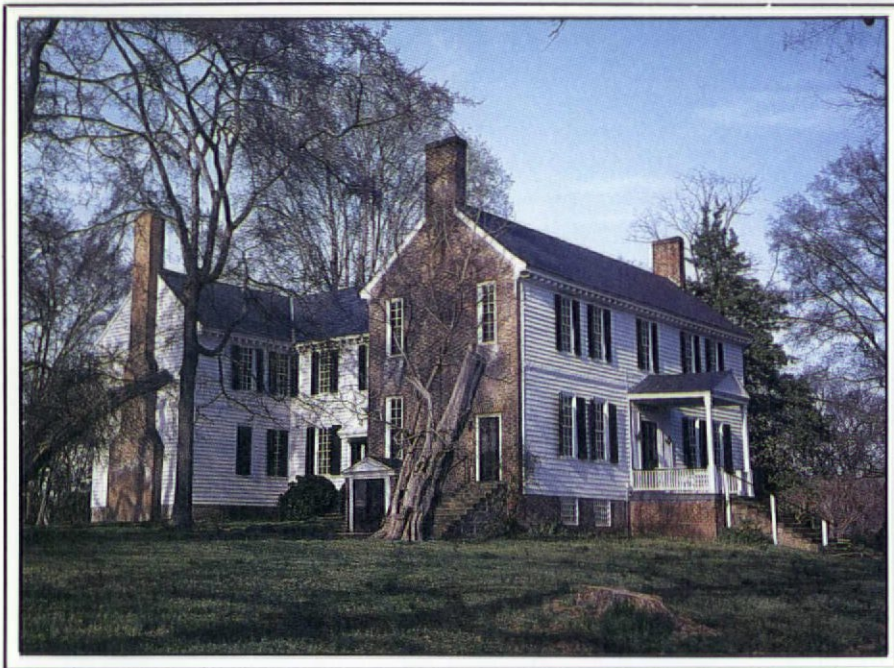
Tuckahoe, Virginia (near Richmond), ca. 1712-1730. A T (the basic shape of the addition) is added to an I (the shape of the original house), making a large H. Note the huge end chimneys.
