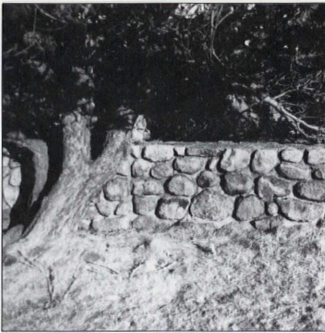
A mortared wall of uniform fieldstones.
