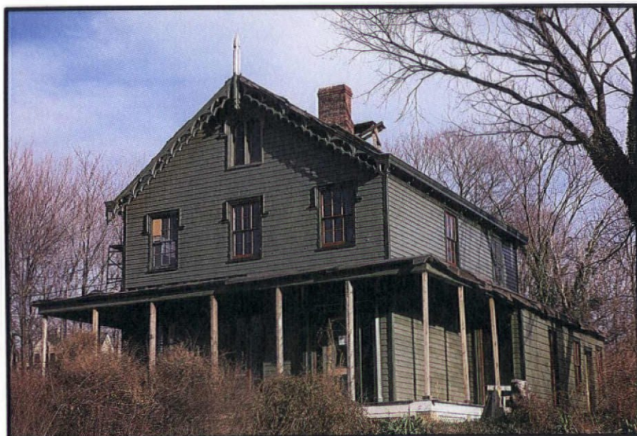
Linseed oil-rich paint has a depth and sheen appropriate for historic houses.
