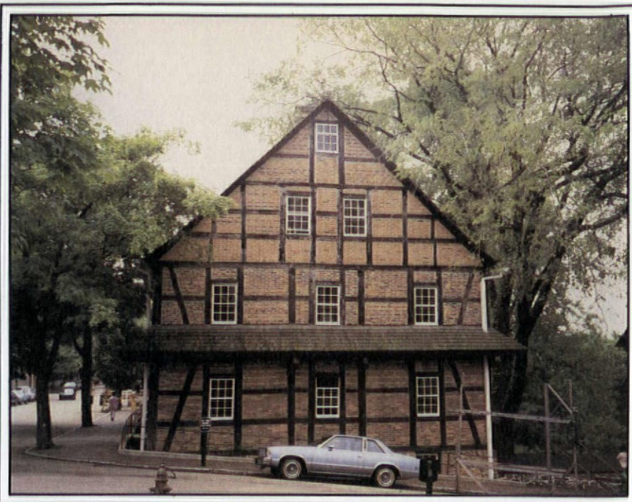
Above: Single Brothers' House (1769) in the Moravian settlement of Old Salem, N.C. This large, half-timbered structure also typifies other German building traditions, including the pent eave above the first floor.
