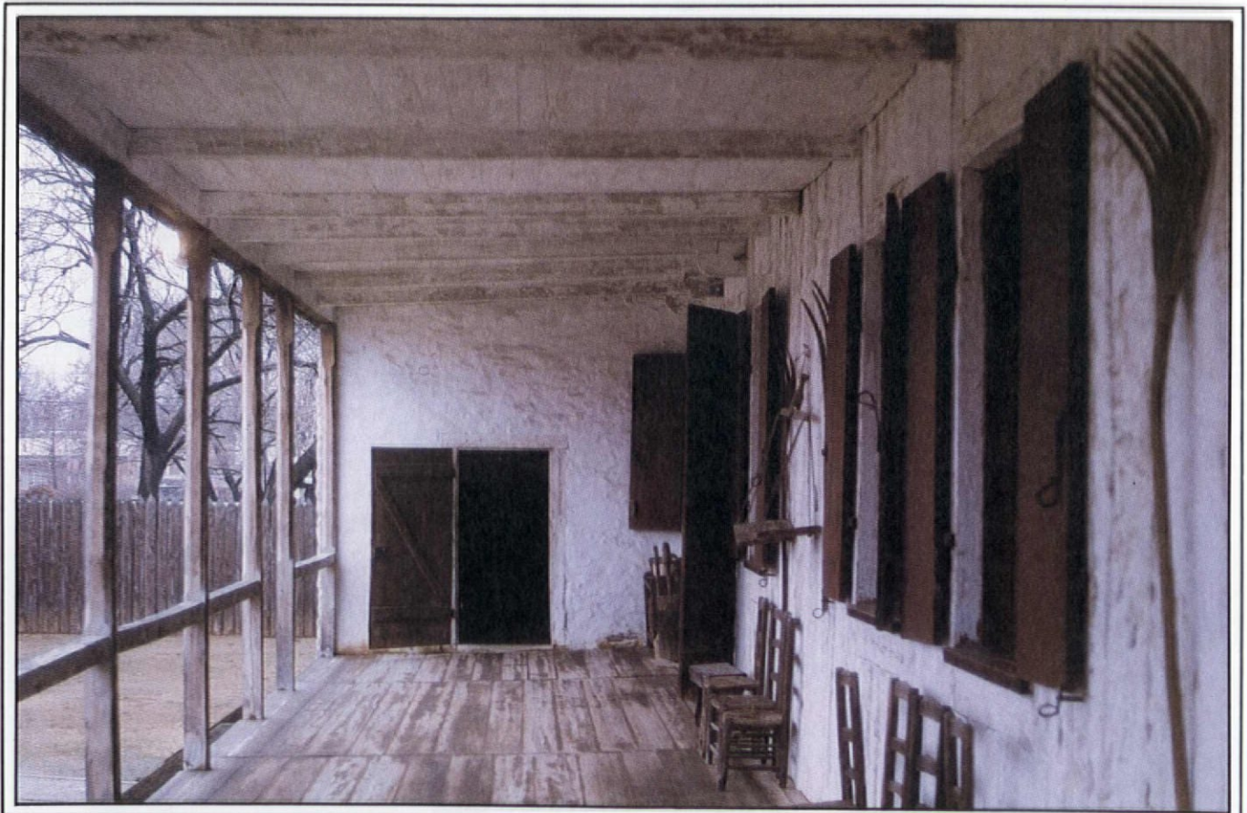
The Bolduc House (c. 1787), in Ste. Genevieve, Mo., has the deep rear porch common to French houses.
