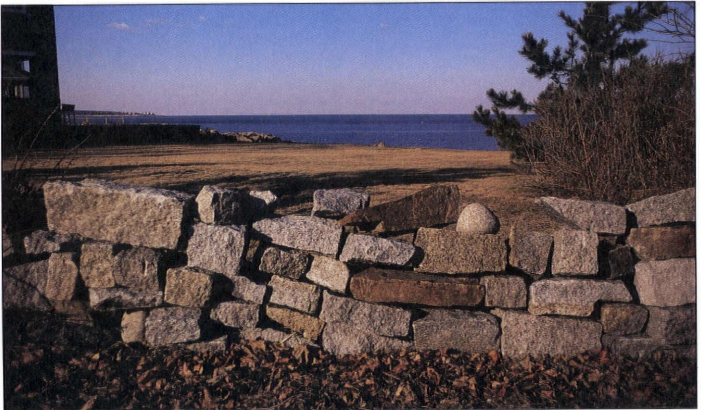
Although not particularly stable, this picturesque pile on the ocean can be easily relaid as it tumbles: The wall is low and the stones are small.
