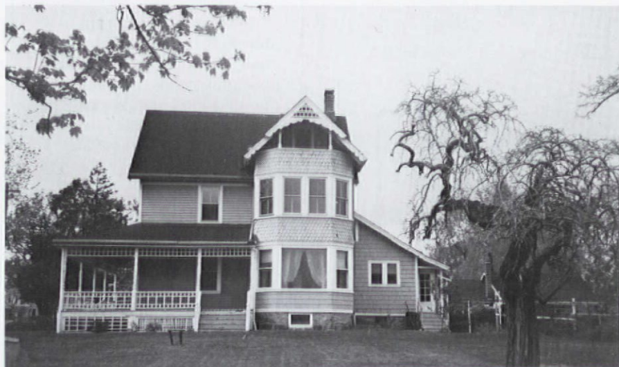
Left: The Gardellas' Stick Style Victorian. The six-sided tower on the side elevation is a little unusual, but the wooden siding and porch detail are typical.
