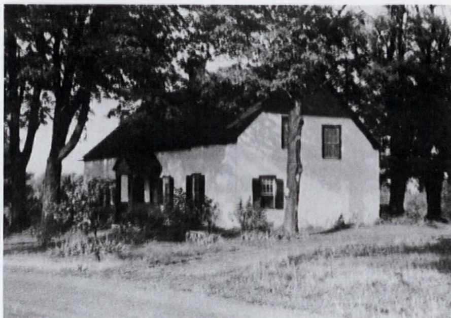
The black T-lock shingles were new when this photo was taken in the 1940s. (The mow door has been replaced by a window.)
