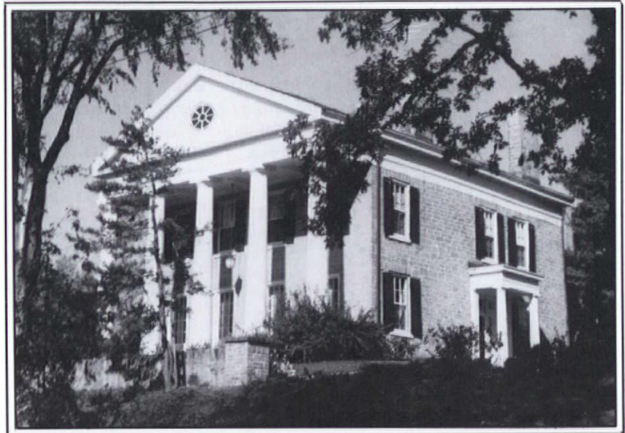
Hays House (1837-38), Marshall, Michigan: The temple form expressed as a portico added to the gable end of a simple rectangular house.
