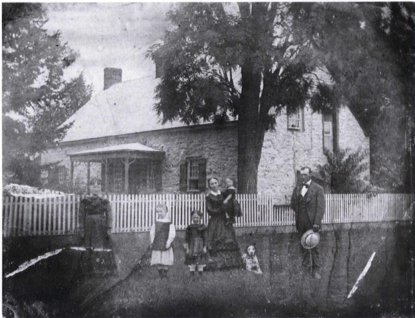
This c. 1880 photo probably depicts the cedar-shingle roof that the author found preserved under the T-lock shingles. (Note that the house is already more than a century old in this photo.) The door on the gable side is a "mow door" through which grain sacks would be thrown from a wagon into upstairs storage. The dormers described in the article are on the back of the house.
