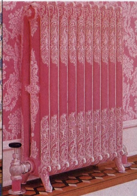
"Painting out" the radiator by matching the wallpaper (American Radiator Co., 1905).
