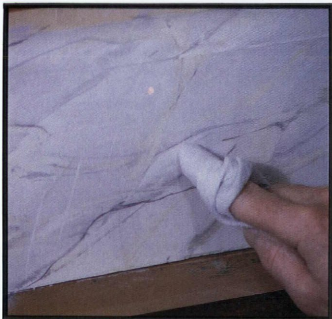
Wiping off the glaze in selected spots exposes some white ground coat, creating "quartz patches."
