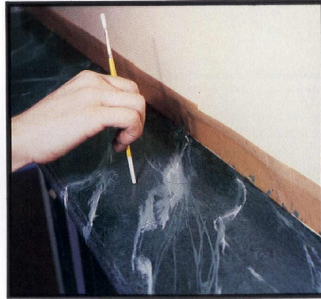
It's possible to draw in hairline cracks with the end of a small brush, toothpick, or even your fingernail.
