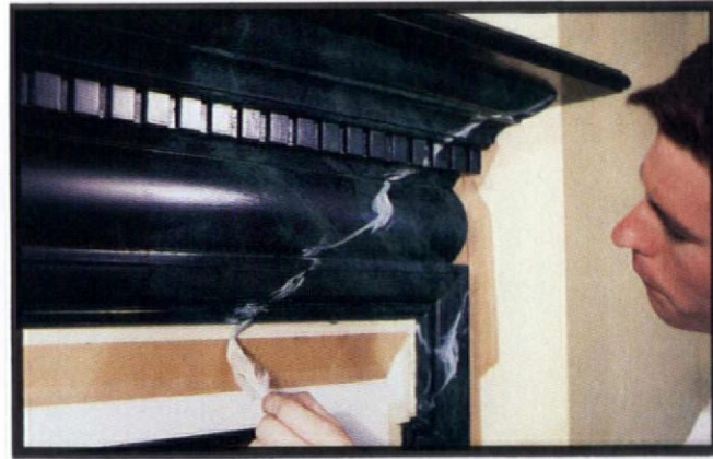
Fine white veins are added, following shadows in the undertone and larger veins.
