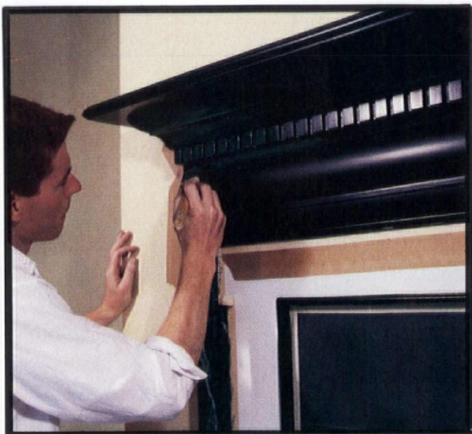
After applying a black ground coat, Jim brushes on the undertone glaze.
