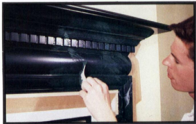
Here, green-tinted glaze is applied with a feather to create broad veins.
