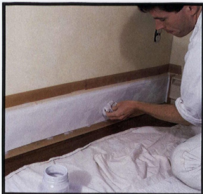
Here, he "busbes" the broad veins with a bunched-up, lint-free cloth.
