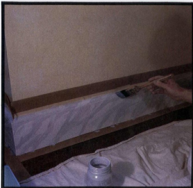
To simulate white marble, Jim applies grey broad veins over a white ground coat.
