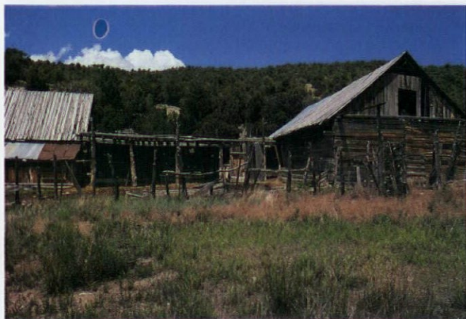
A traditional adobe barn in the center, combined with a "plank" log barn on the right (Los Trampas, N.M.).
