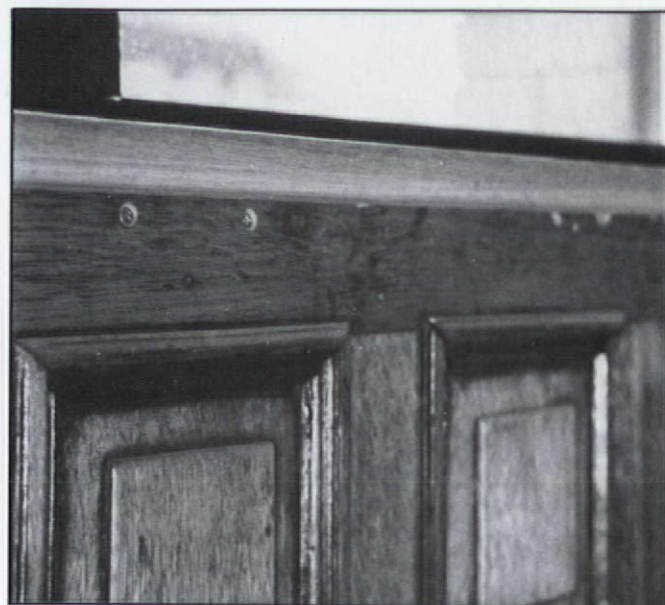
Whole sections of wainscoting that may have to be removed (for access to service areas, for instance) are best attached with screws. These screwheads will be hidden by wood plugs, but they'd be almost as invisible if stained or painted black.
