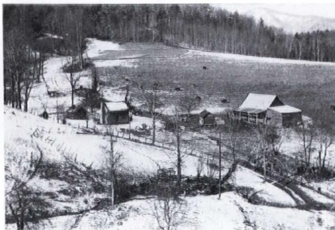
One-pen, windowless log house surrounded by log barns, springhouse, and smokehouse (Iron Duff, N.C.).
