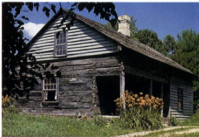
An example of a Norwegian “svalgang” — and integral recessed porch and corner chimney (Dane Co., Wisc.).
