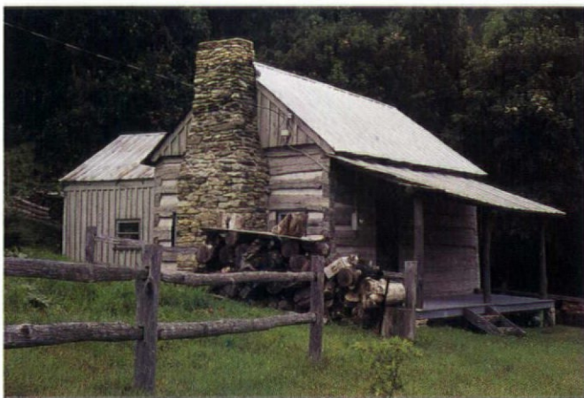
A frame gabled ell added at right angles to a one-pen plan log house (Henson House, Jonas Ridge, N.C.).
