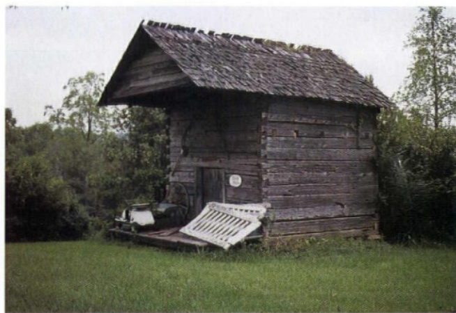
Early 1800s log smokehouse with rare, surviving wood-shingle roof (Burke Co., N.C.).
