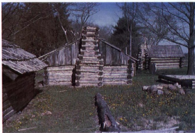
Reconstructed log soldier's butts (Valley Forge, Penn.). Note log chimneys and in the round wall construction.
