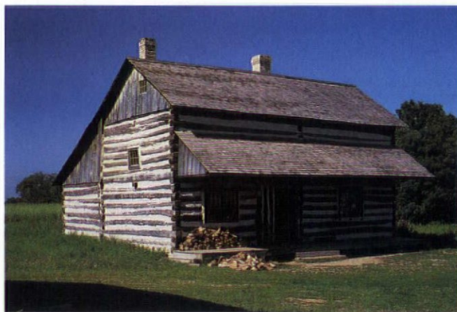
The Turck-Schottler House sports vertical gable boards, a pent roof, and rear shed addition (Old World, Wisc.).
