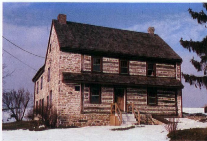
A two-storey log house with rare stone-end construction, restored in 1986 (Chester Co., Penn.).
