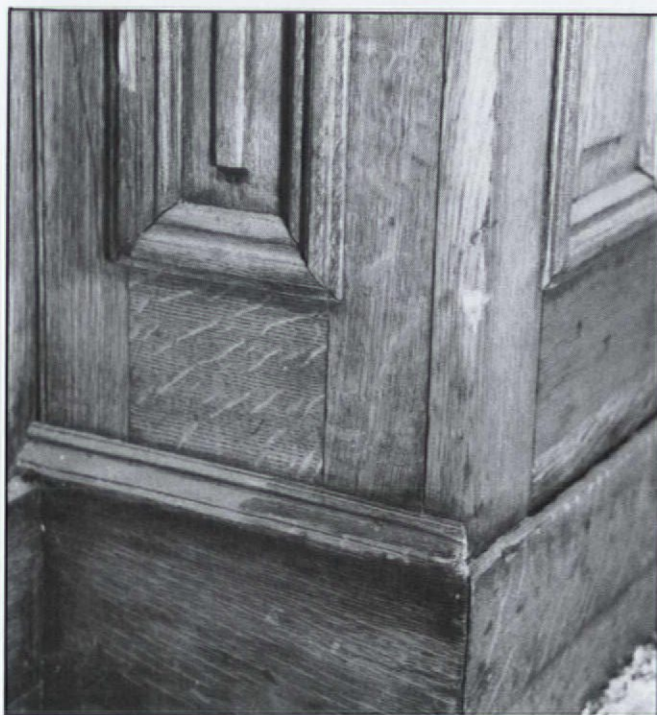
Whole sections of wainscoting that may have to be removed (for access to service areas, for instance) are best attached with screws. These screwheads will be hidden by wood plugs, but they'd be almost as invisible if stained or painted black.
