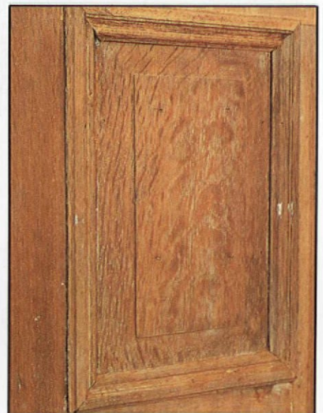
Completed panel was reinstalled with finishing nails, left and right, in pre-drilled holes. The panel floats and should survive another 100 years.
