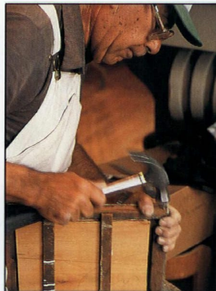
Some mouldings were salvaged, others newly made. All were nailed in the original "picture frame" arrangement that allows panels to move.
