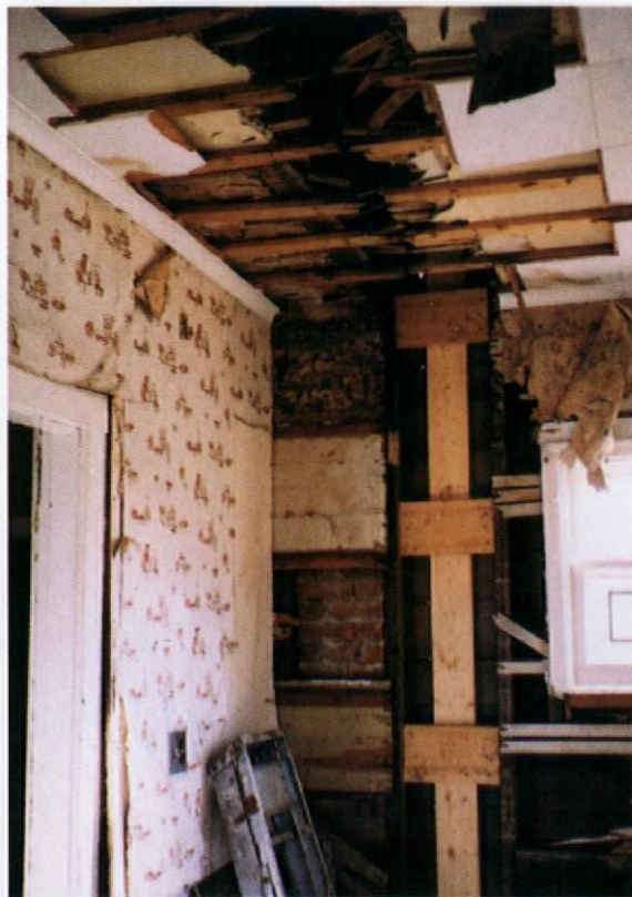
Above: our "mobile bome" en route. Left: Here's how our kitchen looked — note the severed furring — after it was joined to the rest of the bouse.
