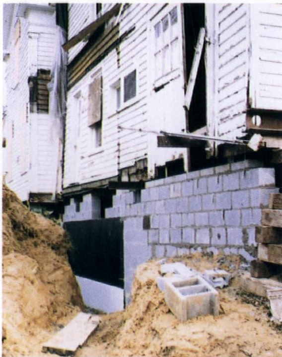
Above: Our half-a-house is met with wholehearted dismay by Betty Lee and my Dad. Left: The foundation of poured concrete and concrete blocks was built up in the hole over which the house was suspended.
