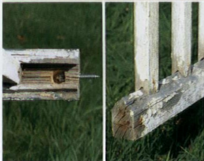
A banger bolt and adapted nut (above) will often double for a true rail bolt. The nut and machine screw fasten the rail through two holes (below left) after the wood screw has been anchored in the support. Foot rails (below right) last longest when constructed to shed water.
