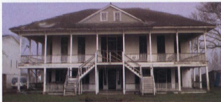
When is a porch not a porch? When it's been enclosed in aluminum siding and perforated with windows (top).
