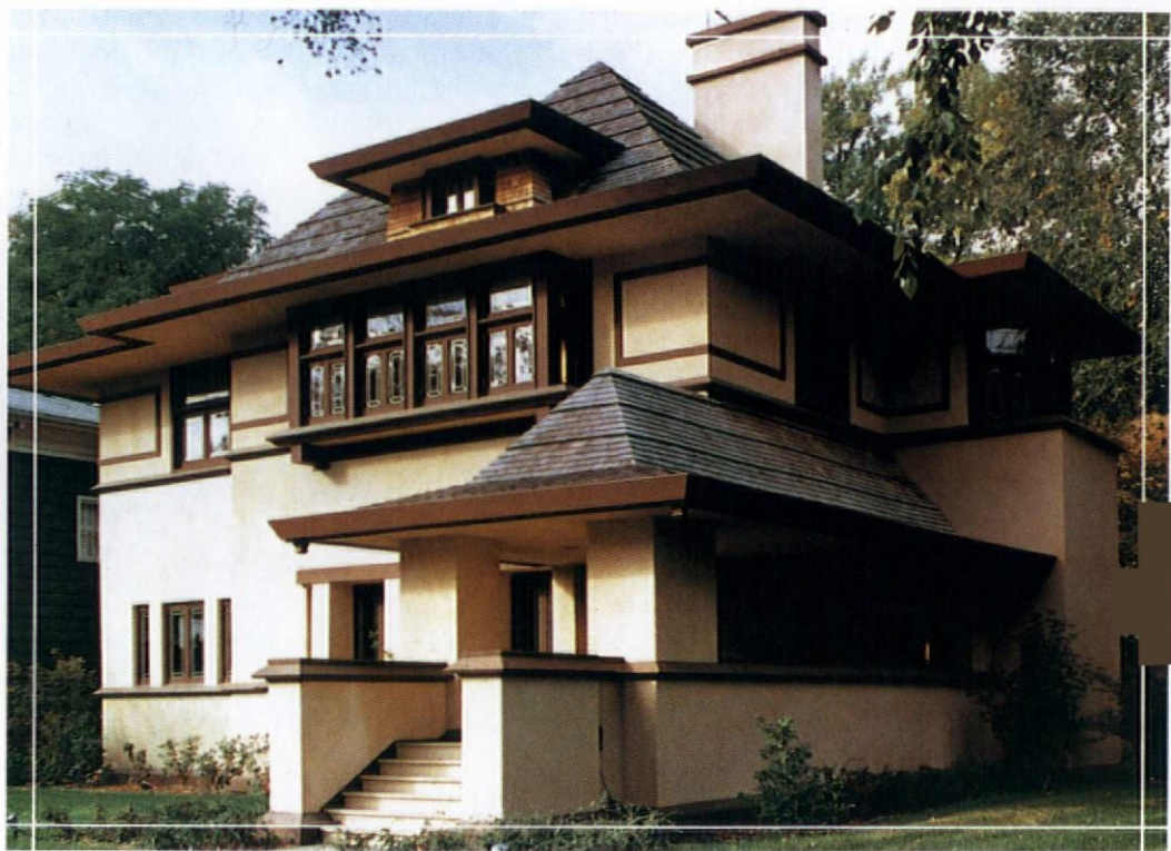
Wood banding on stucco became a favorite exterior treatment of the Prairie School, as seen in Frank Lloyd Wright's Edward R. Hills Residence (1906) in Oak Park, Illinois.
