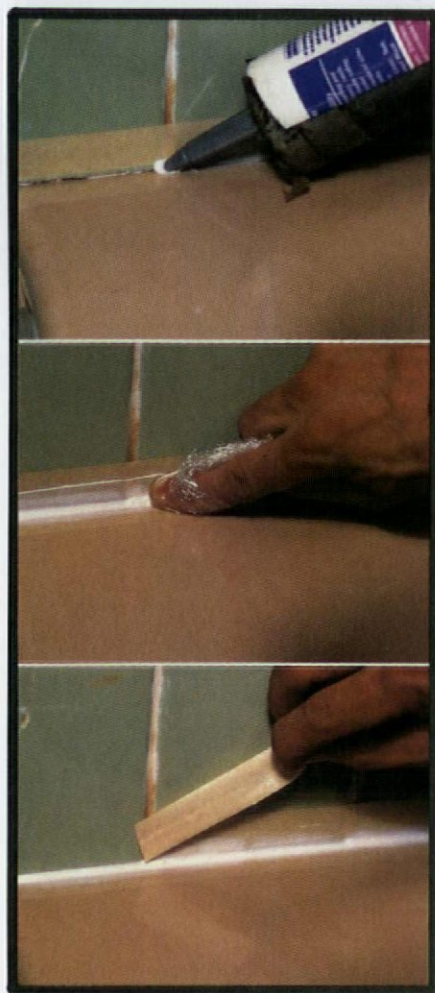
Top: Mask the joint at the appropriate bead size and gun in caulk. Middle: “Tool” the bead so caulk is thinnest where it meets the tape. Bottom: Remove the tape immediately, before caulk skins over (bottom).
