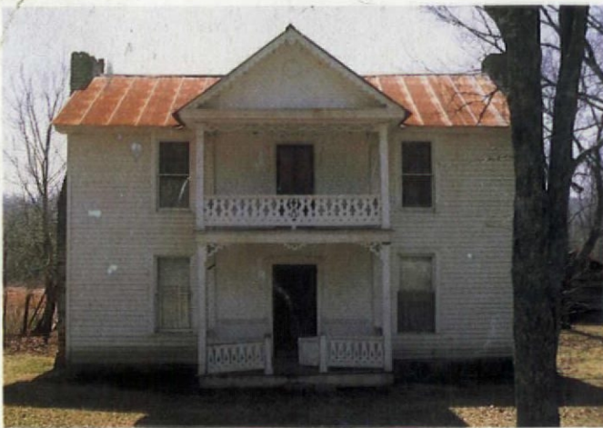
Exterior gable-end chimneys of brick or stone and stone foundations are other features that help identify the Middle Tennessee I-House. Pictured at top, the Bass-Morrell House in Giles County; above, the James Dickson House in Perry County.
