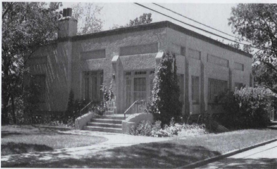
Tar isn't the only solution open to this flat-roofed house.
