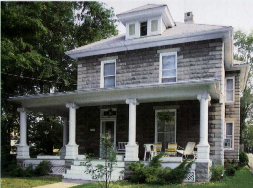
(Top) The classic Homestead in Rebooth, Delaware: tall, narrow (one-room wide), with a plain gable front and front porch. (Above) Located in Winchester, Virginia, this Foursquare uses textured cement blocks.
