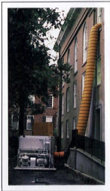
A giant drying machine was used to rapidly remove moisture from Charleston's First Presbyterian Church — with disastrous results.
