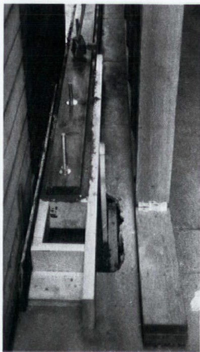
The completed beam with sill attached, still showing the end form.
