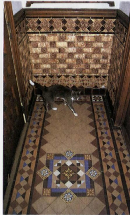
Monochrome-glazed embossed majolica tiles are used for the wainscot in this handsome Haddonfield, New Jersey, vestibule. The floors are of encaustic tiles.
