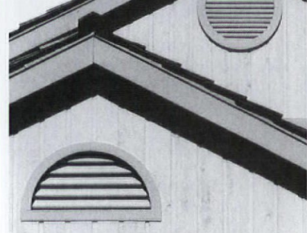
All Sammamish's gable vents have a stout mesh back for insect control.
