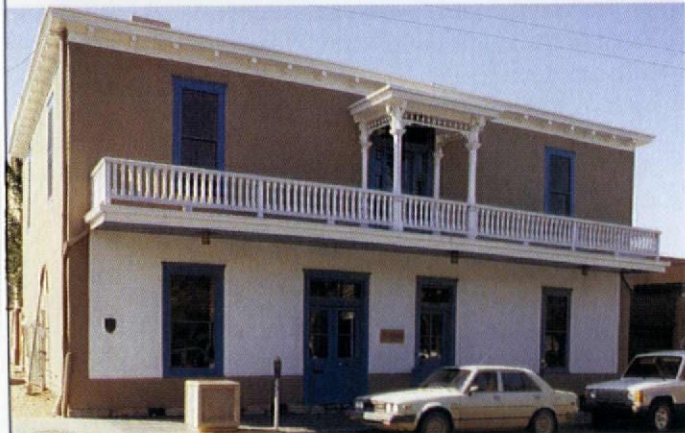
The 1890 Felipe Delgado House, an example of the Territorial style and its effects of fancy millwork and doublehung-sash windows made available by railroad commerce.
