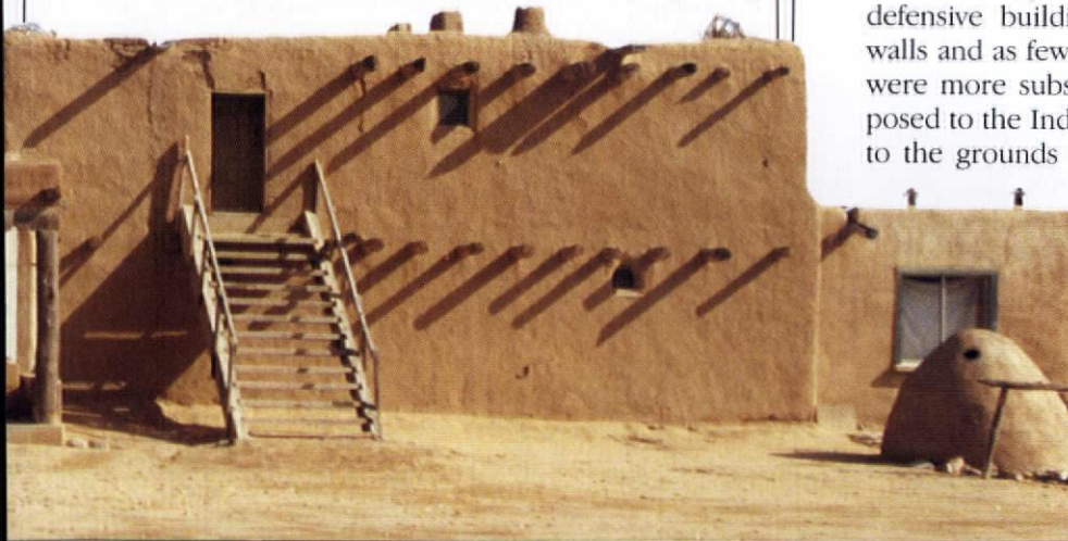
The San Ildefonso Pueblo in New Mexico, a traditional Indian house group dating from various periods. (Note the prominent vigas and set-back second storey.)
