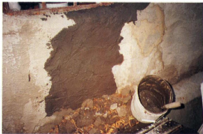
Left: A 1/4-inch application of "slop" dries on the wall. This layer of mud has to be reapplied yearly because it peels off every winter. Right: This wheelbarrow is filled with handmade bricks to rebuild
