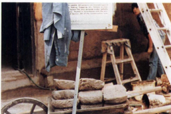
the 6-foot hole. After they were sun dried, I tested their strength by jumping on them. My "stress test" must have been accurate: They're still holding up the wall.
