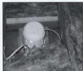
Glass wool batts install readily between framing members. As with all insulation, heat-producing fixtures should not be covered.
