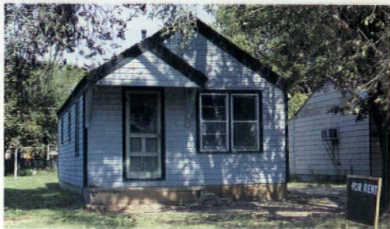
The shotgun's classic proportions (a length two times the width) is often exceeded in Oklahoma, as in this uncommon hipped-roof example (top). Substitute siding and new windows complete the modernization of this shotgun (above). One of the few shotgun houses (below) that still displays original board-and-batten siding.
