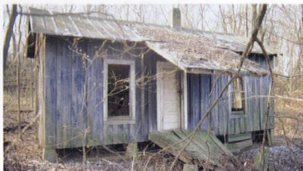
Only battens were used to close in the planks of this "box frame" house near Ripley, Tennessee.
