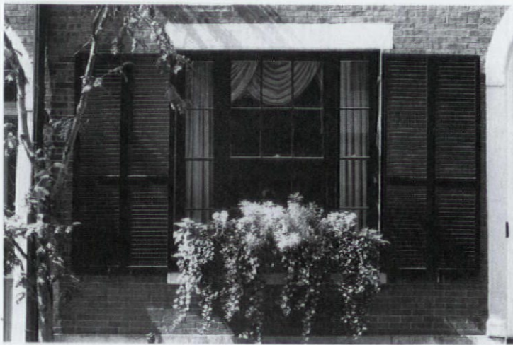
These unusual double-width blinds may have been installed to shield carpets, paintings, and delicate textiles from sunlight damage.
