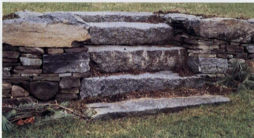
A finished retaining wall, complete with large capstones and granite steps.
