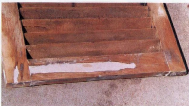
(above) The horizontal edge of the hinge retarded drainage, and condensation behind it contributed to wood rot. When it was necessary to add to previously hardened filler (below), we roughed up the surface thoroughly with a knife or nail and coarse sandpaper.
