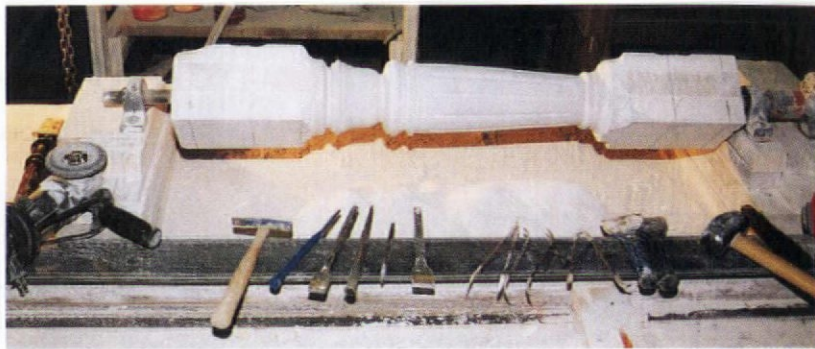
Detail work on balusters with ornamental contours is done by hand with chisels, rasps, and a grinder.
