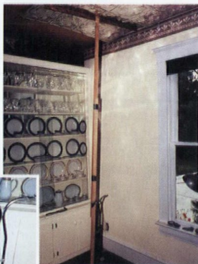
A pogo stick T-brace is easy to assemble, adjust, and move around a room.
