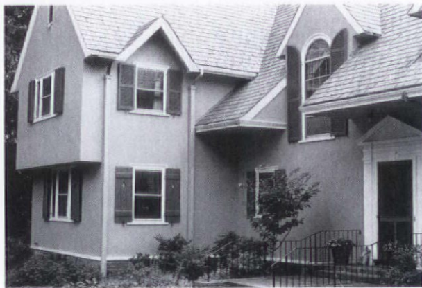
Blinds became common for second-floor ventilation, while solid shutters maintained privacy and security below.
