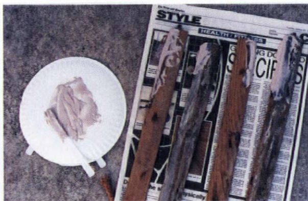
Several vanes in our shutters had lost corners or chunks, or were cracked down the middle. We successfully "glued" cracks together, and rebuilt missing parts with the resin. We added filler and filed, again and again, until the original shape was achieved.
