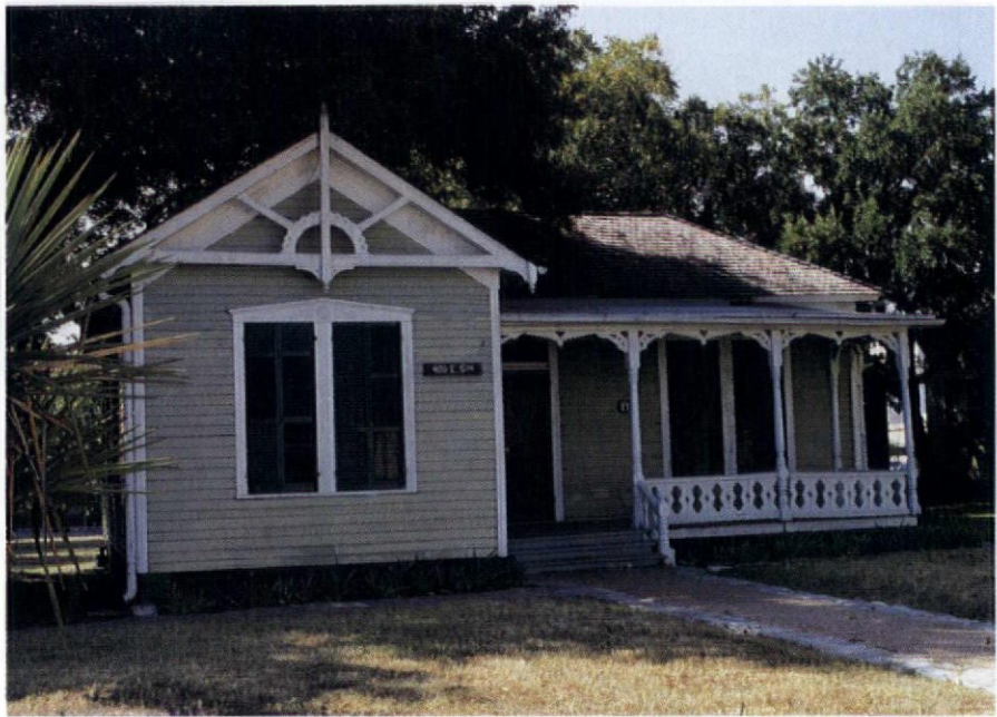
The 1890s home (above) of short story writer O. Henry in Austin, Texas, is a handsome "box frame." Suggested improvements included adding a thin space under the siding (right) for insulation.
