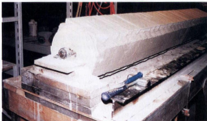
At first, it is faster to saw and chisel off high points to achieve the rough-round cylinder (note reference circle drawn on end).
