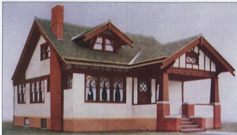
Note the horizontal floorplan and the low-pitched gable roof on this early 20th-century bungalow.
