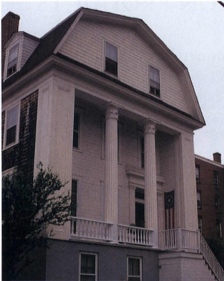
(above) The clues were there: Notice how the utilitarian staircase clashes with the formality of the columned porch. (inset) A twin structure shows how the Big House looked before the alterations.
