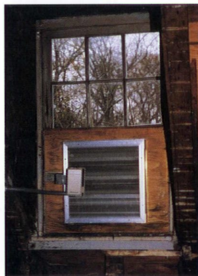
Where power is available, humidistats (the box here) can monitor interiors to activate ventilating fans.
