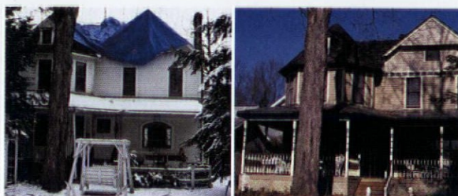
Once, ugly blue tarps covered a hole in the roof (left). Now, the house sports a five-color paint scheme (right).
