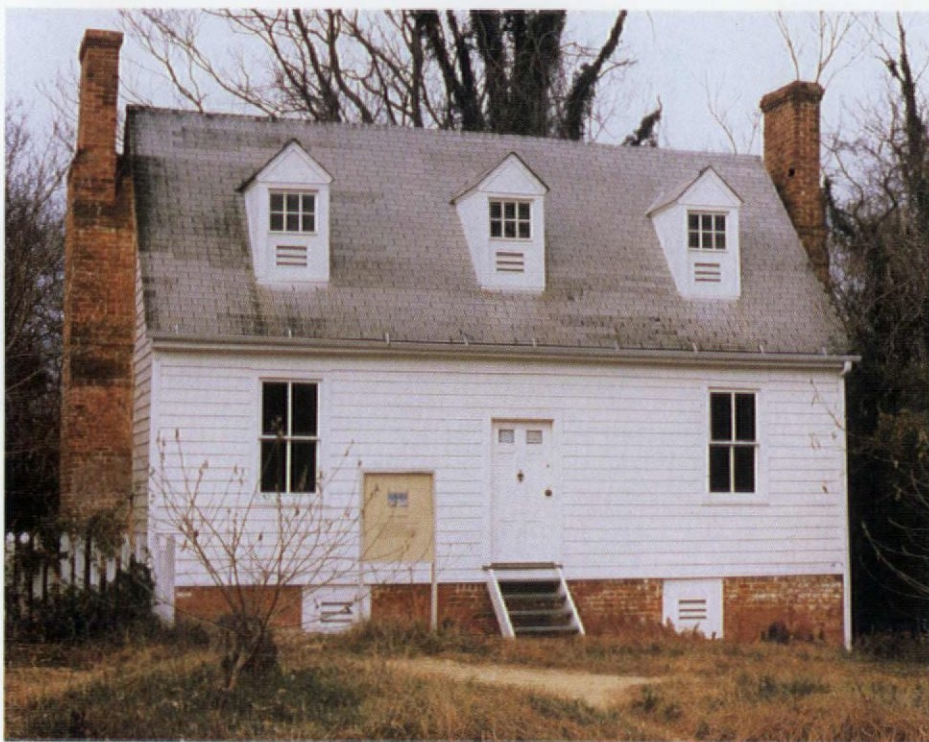
Attic and basement window vents allow air circulation in the mothballed Booker Tenement in Williamsburg, Virginia. Vents are substantial wood-louver construction that deflect water and resist tampering.
