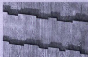
Asbestos-cement "Thatch Butt" shingles.
