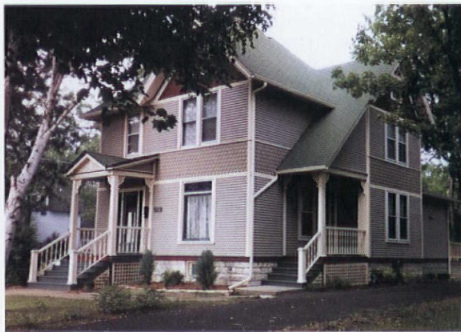
Stripping the wide, monotone, asbestos-cement shingles from this 1886 Queen Anne in Wheaton, Illinois, revealed little moisture damage but plenty of nailholes. Repairs included replacing missing trim boards, and cracked shingles and clapboards. Well-protected by new paint, the house will soon receive a plaque from the city historical society.
