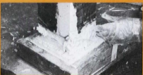
...were completely sawed off and replaced with...
