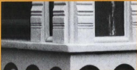
...sanded, nailed, stained or painted.
