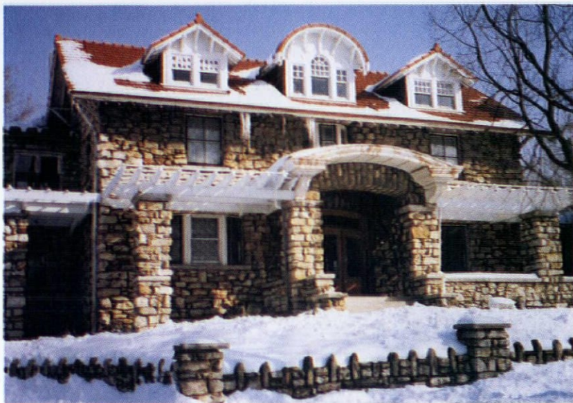
The Rigbys' stone house in Kansas City, Missouri, exhibits a combination of influences, including Craftsman and Colonial Revival. Note the decorative rafters that form a pergola porch across the building, a popular Arts & Crafts feature.
