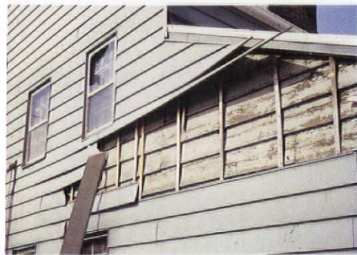
Furring strips are commonly used to level a wall under aluminum siding.
