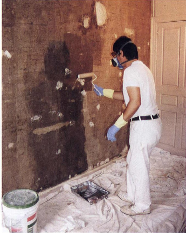
Peter applied our consolidant mix in three coats, using a bristle brush for edges and a roller for fields.
