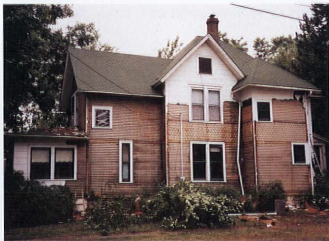
Stripping the wide, monotone, asbestos-cement shingles from this 1886 Queen Anne in Wheaton, Illinois, revealed little moisture damage but plenty of nailholes. Repairs included replacing missing trim boards, and cracked shingles and clapboards. Well-protected by new paint, the house will soon receive a plaque from the city historical society.
