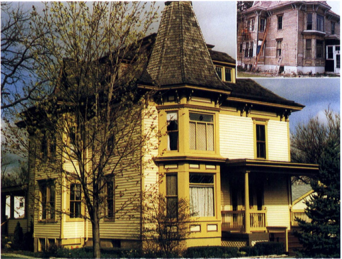
The 1887 Conrad house (above), modernized ten years later with a mansard roof, tower, and two leaded-glass bay windows, as it looks with a 1992 paint job. Early outdoor work (inset): Removing a century of peeling paint.
