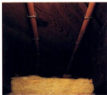
Rubber hose with an internal barrier (above) can be stapled up. Note the air space before insulation. The oxygen barrier is inside the wall (below).
