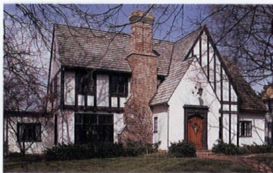
The steeply pitched double-gabled front and massive front-facing chimney appear again on a typical English Revival house in Kansas.
