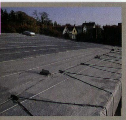
Top: Moisture condensation and ice dam leaks have blackened this attic with mildew and now feed fungal growths. Above: Heating cables — a popular but dubious ice dam cure.
