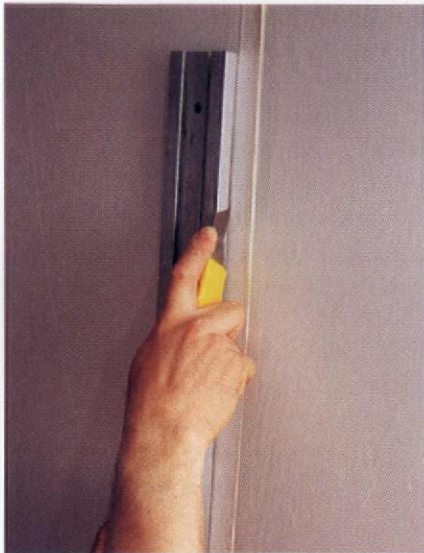
Hang canvas or fiberglass liner so that one sheet overlaps the other. (Left) Double cut using a long straightedge to make seams seem to disappear.
