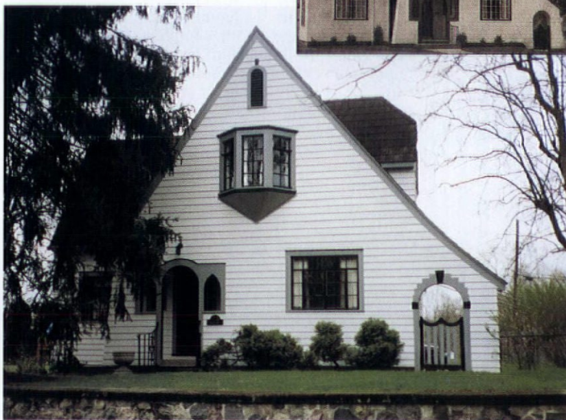
Double vision: The c.1930 Dyer home (above) is an exact match for "The Crestwood" house plan in the 1928 Home Builders Catalog (inset).
