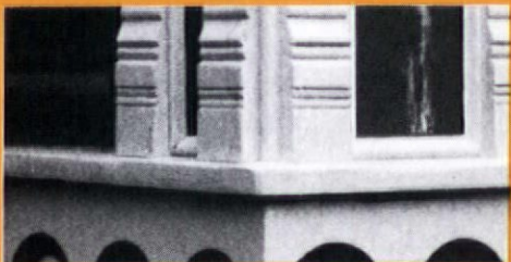
...sanded, nailed, stained or painted.
