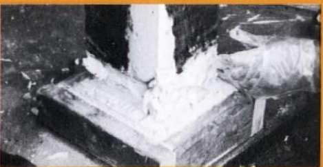
...were completely sawed off and replaced with...
