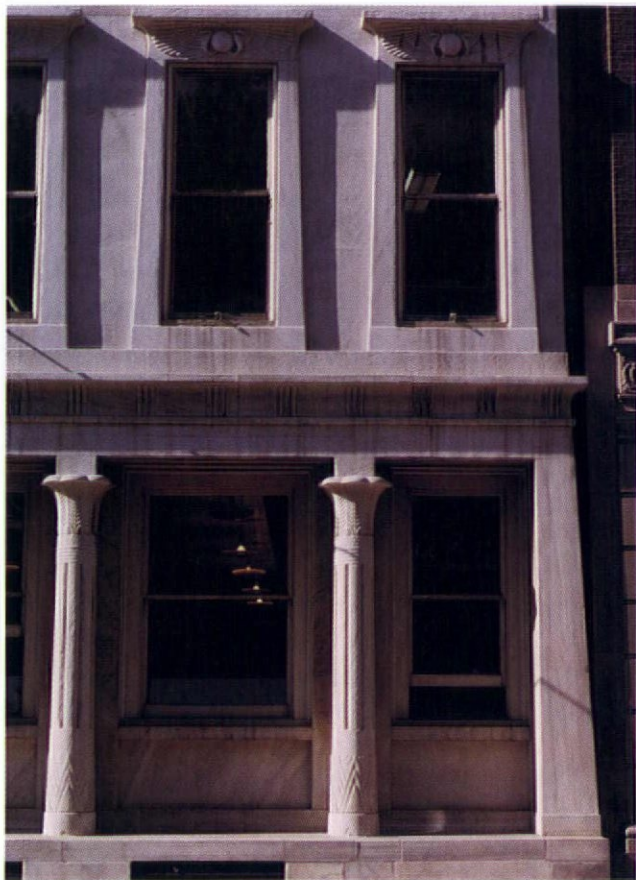
Pennsylvania Fire Insurance Company, Philadelphia, Pennsylvania (1838; John Haviland, architect). Although built as offices, this small, narrow, four-storey, party-wall structure is more domestic than commercial in feeling. Note its many Egyptian-style details.
