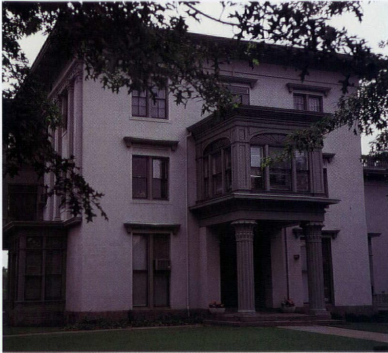
Elizabeth Athorp House, New Haven, Connecticut (1837; A.J. Davis, architect). This Italianate mansion has an Egyptian entry porch. The second-floor enclosure is modern.
