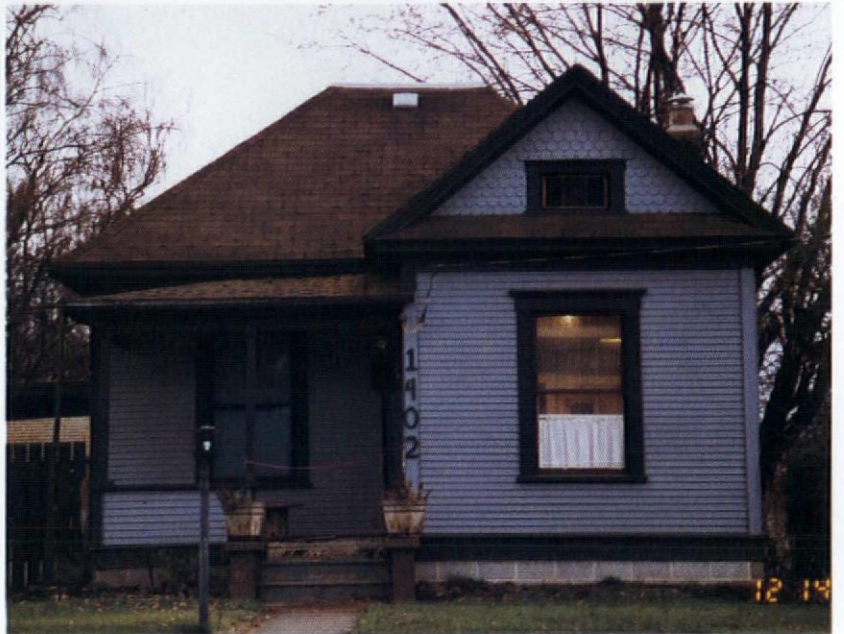
The front of the Nixon's cottage clearly shows the flat top of the hipped roof and the triangular pedimented gable.
