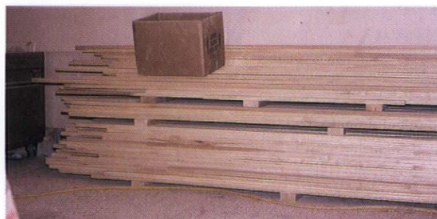
Above: Good stickering gives new flooring plenty of support and air circulation for acclimating. At left: Typical tongue-and-groove flooring features.
