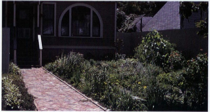
The time-worn, old brick of the herringbone pattern walk looks as if it was laid a century ago. However, the new path is slightly wider than the original.
