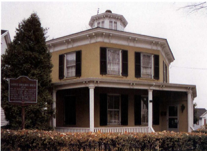
Based on Orson Fowler's model, this 1854 octagon in Boonton, New Jersey, was built with walls of slag concrete that used waste from the town's iron furnace as aggregate.
