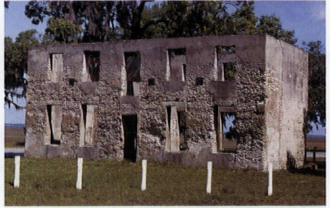
Only the tabby walls of the 18th-century Horton House on Georgia's Jekyll Island survive. This oyster-shell concrete was common in early coastal settlements of the United States.
