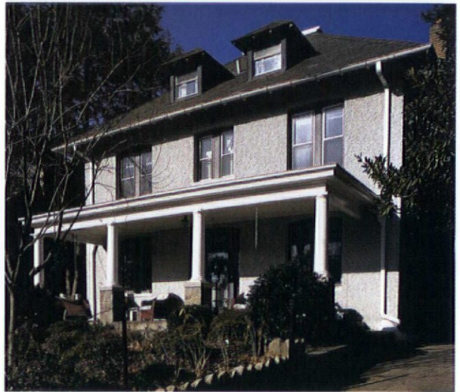
This early 20th-century thoroughly fireproof Foursquare in Washington, D.C., features an interior frame and floors of reinforced concrete; walls are load-bearing tile clad with stucco, easier to use than poured concrete.
