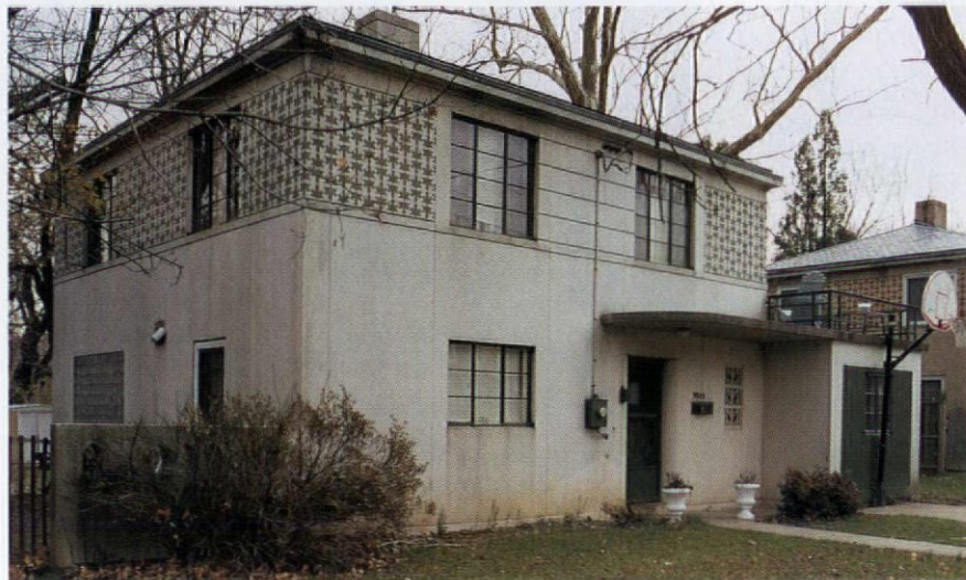
Designed by J. R. Kennedy, this 1935 concrete house in Silver Spring, Maryland, features ornament precast by the Early process.
