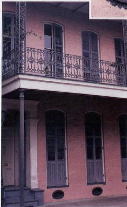
Cellar vents are a common sight at sidewalk level in New Orleans, an old — and effective — response to the high watertable.
