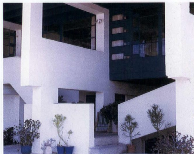
Rudolph Schindler used massive exposed concrete frames to lift the living area of the 1925–26 Lovell Beach House for privacy and an enhanced view of Newport Beach.
