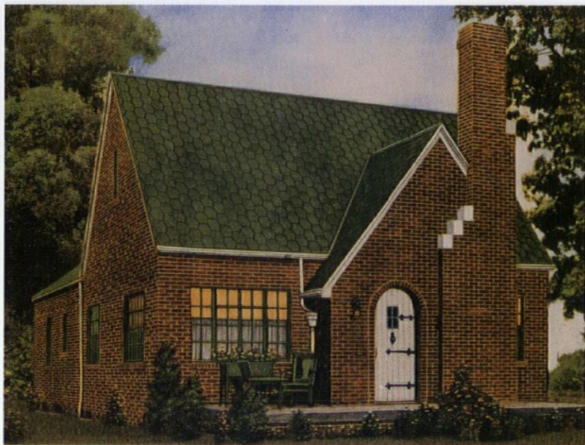
A "colorful asbestos roof" helped ads sell houses in the 1920s and '30s. These black, red, green, brown, and grey shingles can be revived with latex paint.
