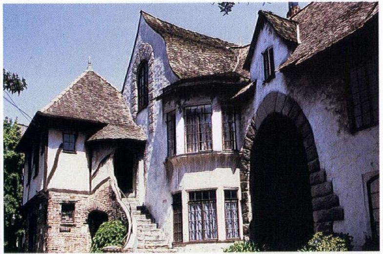
“Normandy Village” in Berkeley, California (1924), combines randomly bonded brickwork, rough-cast stucco, and stone arches for highly theatrical — but far from unique — picturesque effects.
