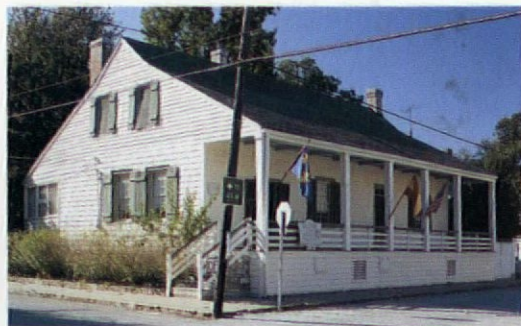
Also in Ste. Genevieve, the Guibourd-Valle House (c. 1807) is an example of poteaux-sur-sole construction. Clapboards were a typical later addition.
