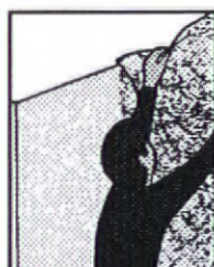
9. Apply mat to 2nd area, overlapping by 1".
