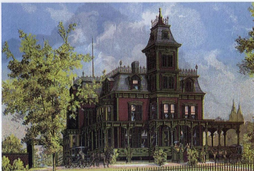
One example of a Victorian mansard roof. The center square tower is not atypical. (Devoe Paint Co., 1885)
