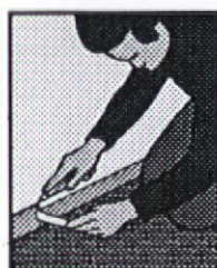
5. Trim mat at baseboard and window.
