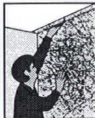
4. Trim excess mat where wall meets ceiling.
