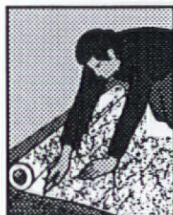
1. Cut fiberglass mat 2" longer than height.
