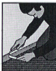
5. Trim mat at baseboard and window.
