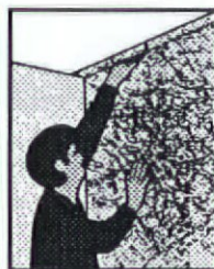
4. Trim excess mat where wall meets ceiling.
