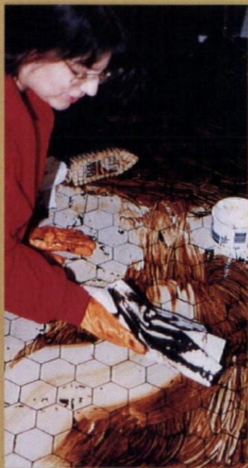
Wiping away linoleum mastic.
