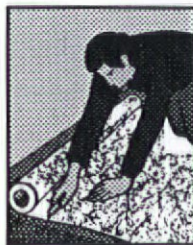
1. Cut fiberglass mat 2" longer than height.
