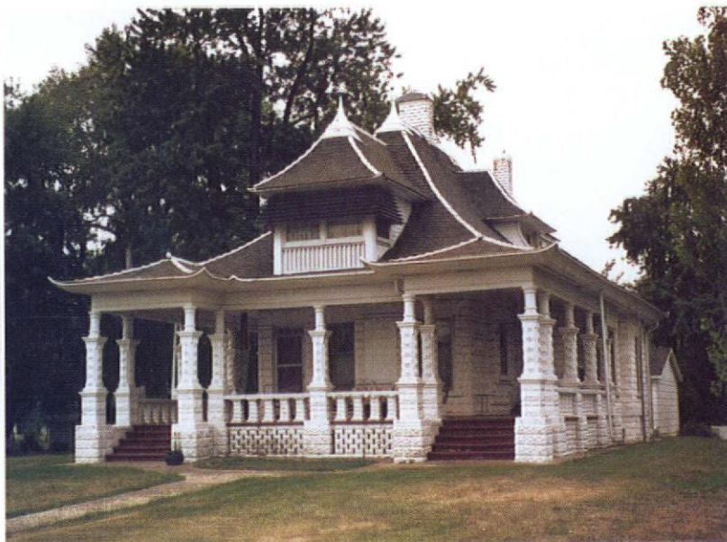
Bungalows found a kindred medium in concrete block. This example, a regional favorite in White Hall, Illinois, takes the "airplane bungalow" to new heights with an uninhibited mix of ornamental patterns.
