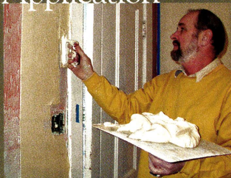
APPLY plaster to the wall from the bottom up; work efficiently (you'll have a 30-min. window).
