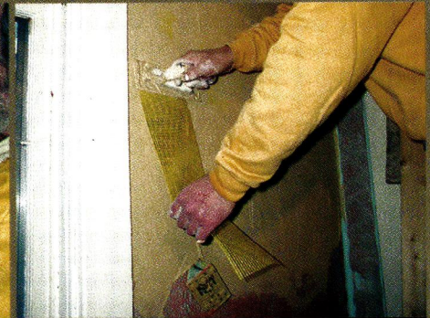
OVERLAP mesh over cracks for added insurance, then overplaster completely.
