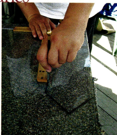
LEFT TO RIGHT: Using a rotary tool with a 1" circular blade attachment, carefully cut the old lead joints halfway through. To cut new panes, score glass with the glass cutter, holding it firmly and using a straightedge as a guide. Then, snap down along the score line with breaker pliers.
