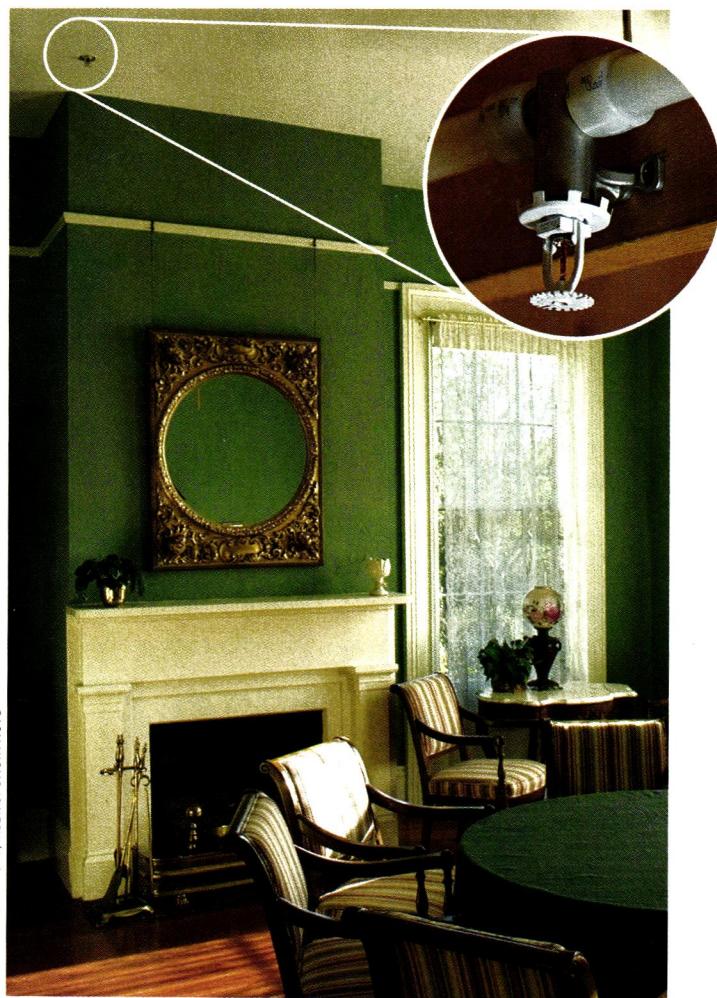
The Brokaw-McDougall house in Tallahassee, Florida, installed a fire sprinkler system with flexible PEX tubing during renovation.
