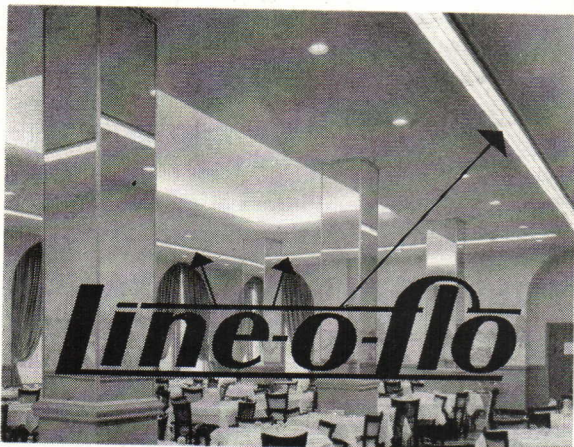
Illustration of continuous-strip "LL" LINE-O-FLO units with lights in the ceiling of a hotel dining room.
