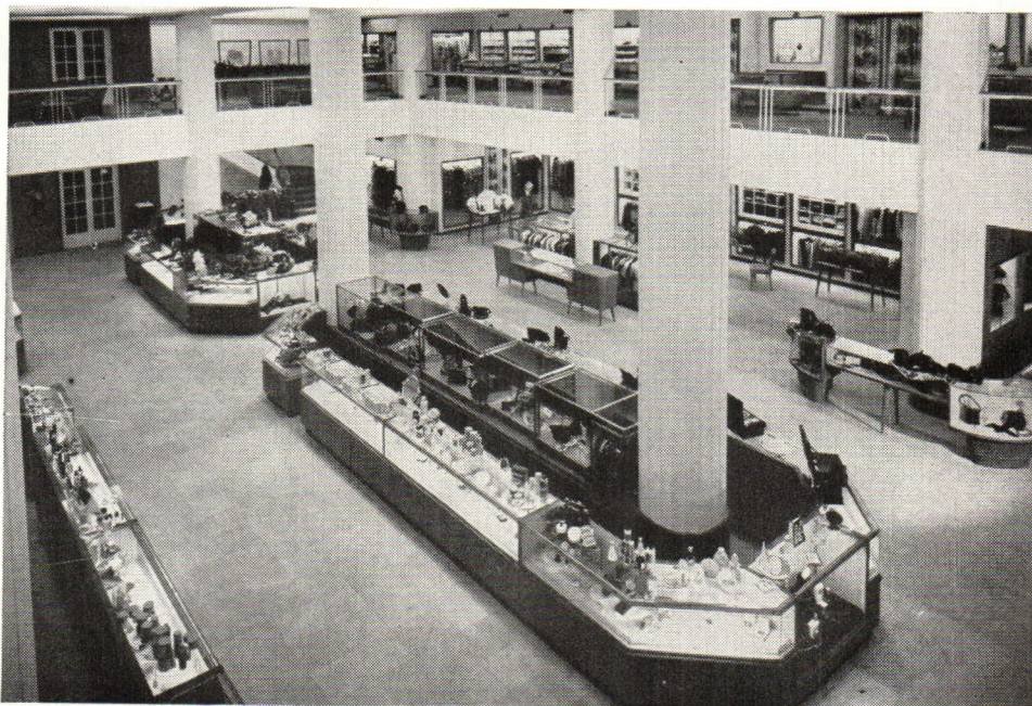
Air Conditioning by Natkin & Co., Houston, Texas.
