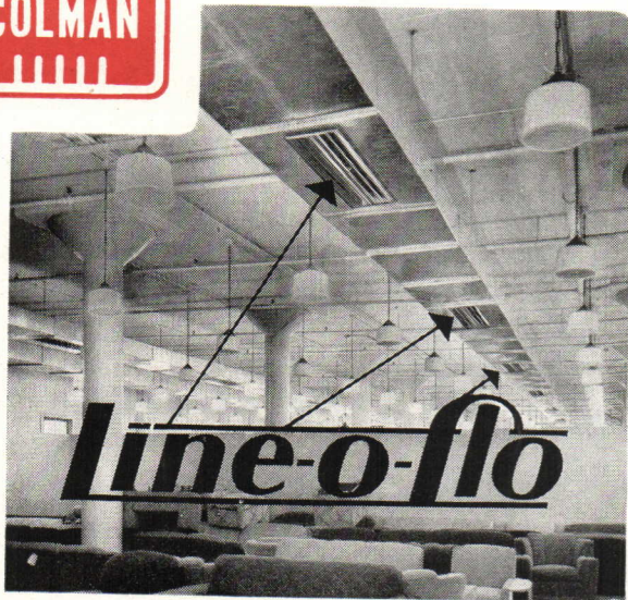
Illustrating use of individual "LS" LINE-O-FLO units set into exposed ducts in a large retail store and show room.
