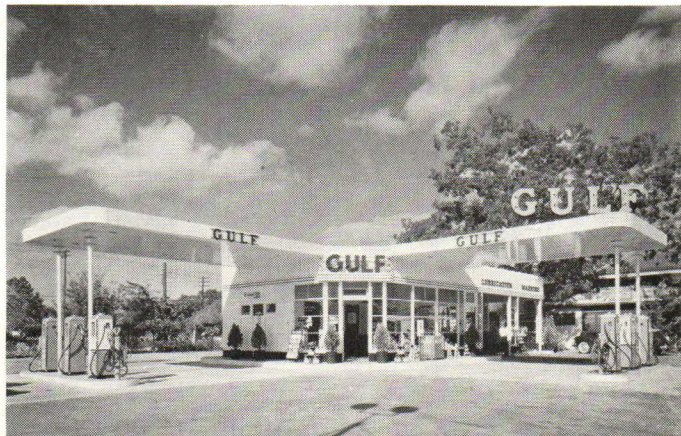
Porcelain-enameled light steel in an automobile service station; one of many applications common today; Steel Building Division, Globe-Wernicke Co.
