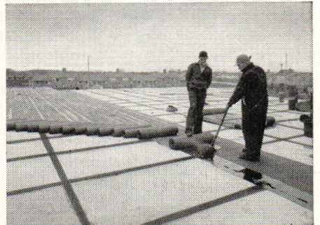
Asphalt roll roofing applied over Cemesto. Pittsfield Township School, Washtenaw, Mich. Architect: C. Nobel. Contractor: DeKenning Const.
