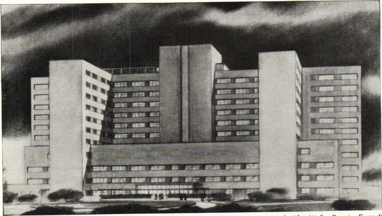
G. M. S. Veterans Hospital, Omaha, equipped with 1,659 fine Fenestra Fenecraft Windows. Architect: Ellerbe & Co., St. Paul, Minn. Associate Architect: Leo M. Daly, Omaha; Contractor: Peter Kiewit Sons Co. & Associates, Omaha.
