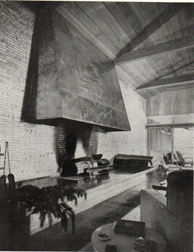
Left: the raised living room fireplace with its ceiling-height copper-hood heater (see Selected Detail, page 89).
