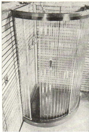
Left: White translucent corrugated sheets serve as doors and walls in these toilet booths. Center: Shower stall walls and curved front are clear corrugated sheets; base is in translucent form. Right: Plastic entrance door has advantages in weight, safety, and cost.
