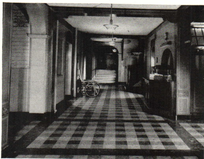
This hospital corridor is typical of the many commercial areas where asphalt tile can be used to advantage. It is a low-cost, long-wearing floor that is easily maintained. Because it is laid one tile at a time, it offers unlimited floor design opportunities.
