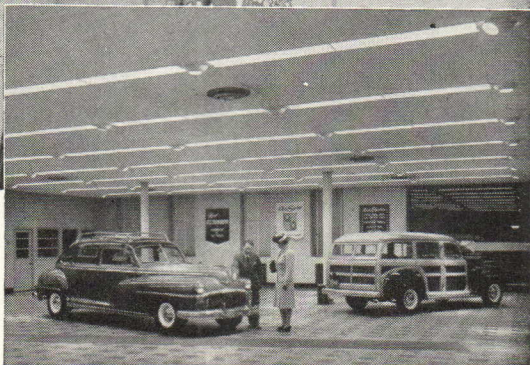
Wiley Recessed Troffers Combined with "Spots" in continuous runs.
