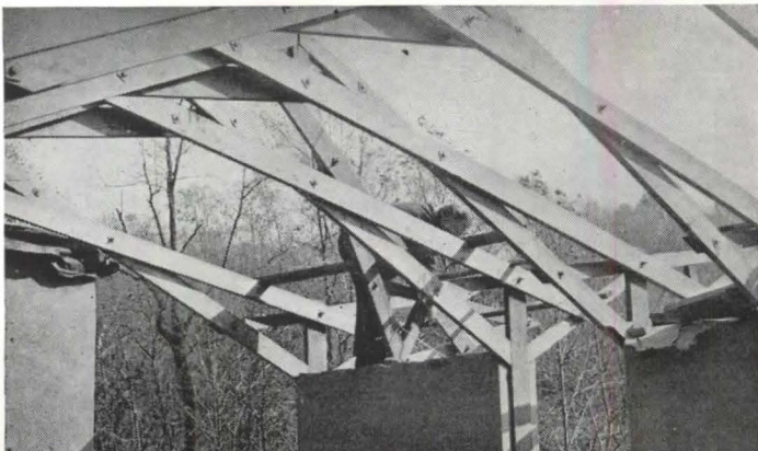
A plan of the roof frame (top, above) shows the spacing of the trusses which corresponds with the three-ft module floor plan, while the positioning of the trusses and the location of split-ring connectors are shown in cross section (above) and photo (left).
