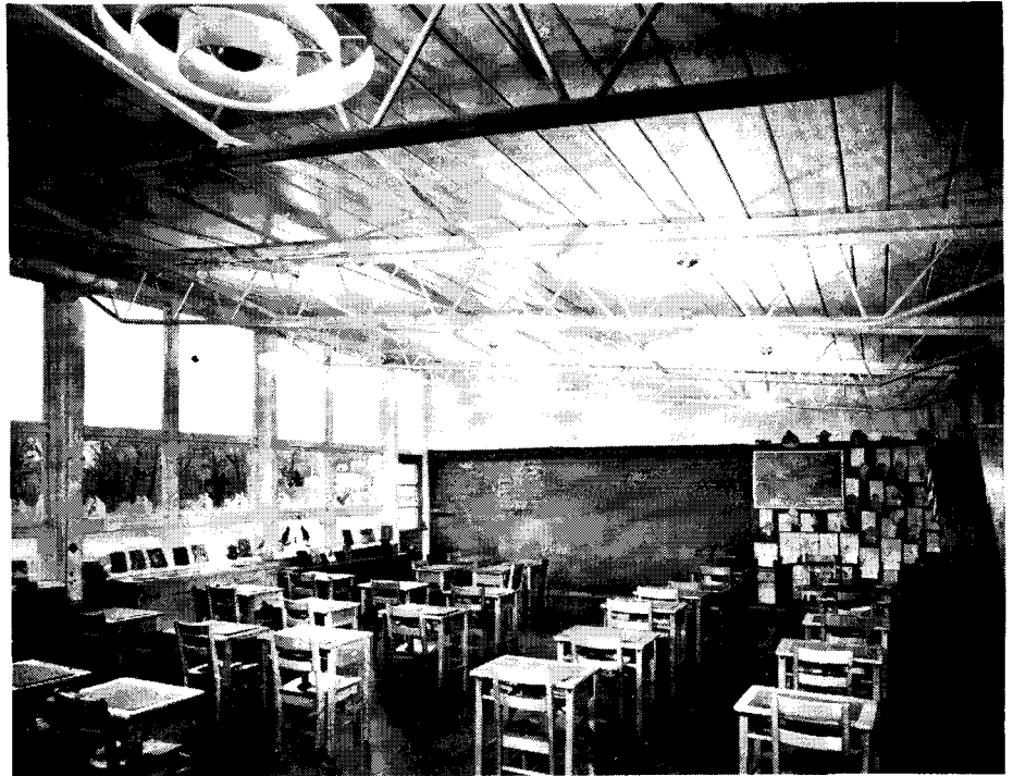
In the typical side-on classroom, the open-web joists are transverse to the room and supported on exposed steel columns. This is a room on the south-east side of the building.
